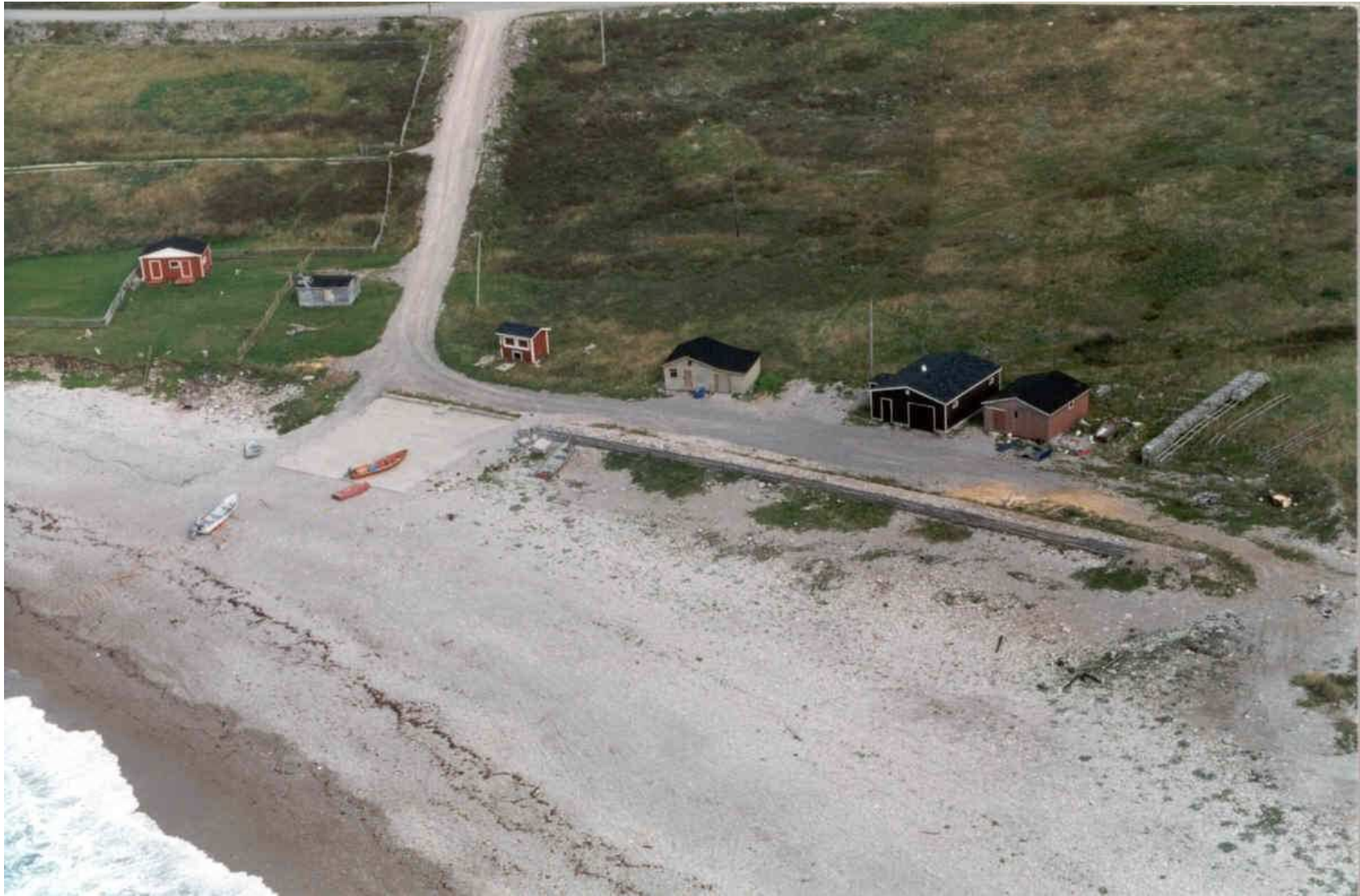
Site Photograph: Aerial View of Ship Cove beach levelling site.
