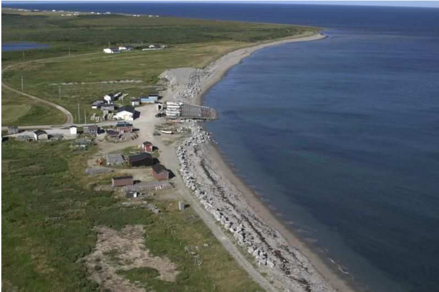
Site Photograph: Aerial View of Black Duck Brook dredging site.
