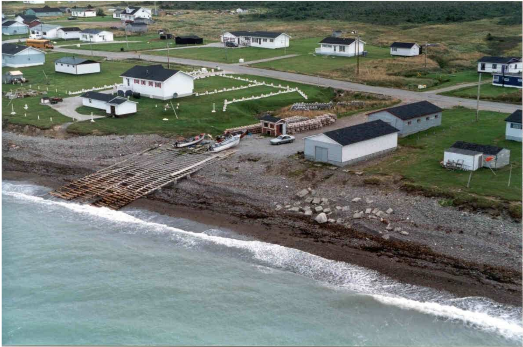
Site Photograph: Aerial View of Mainland beach – Anatole’s Landing beach levelling site.
