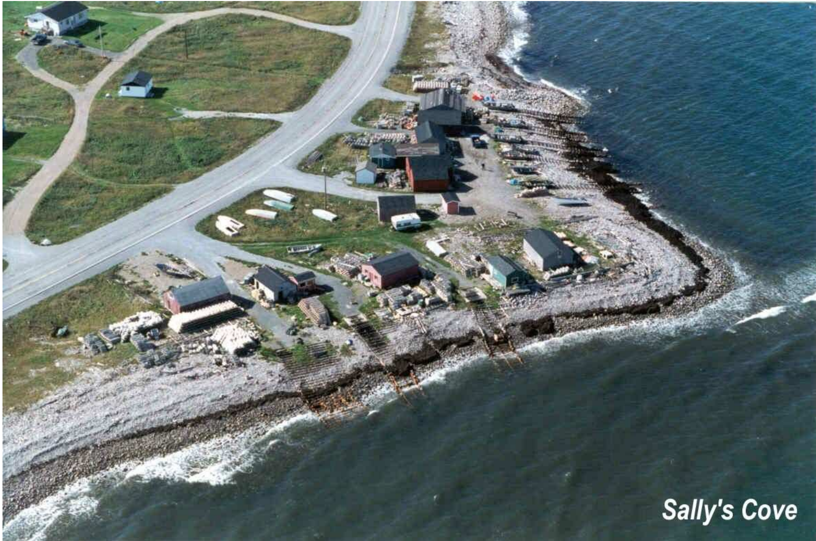
Site Photograph: Aerial View of Sally's Cove dredging site.
