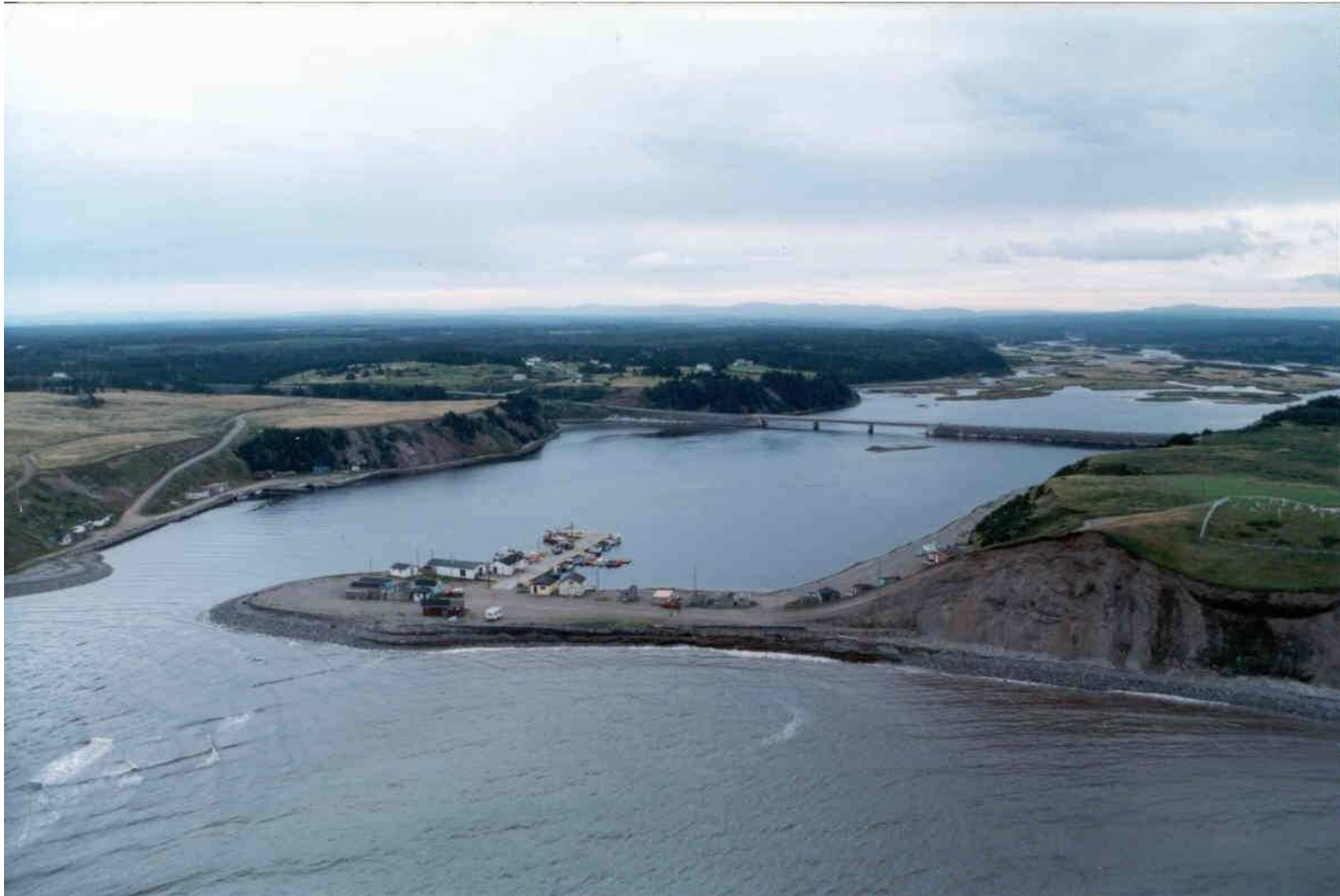
Site Photograph: Aerial View of St. David's (Crabbes River) dredging site.
