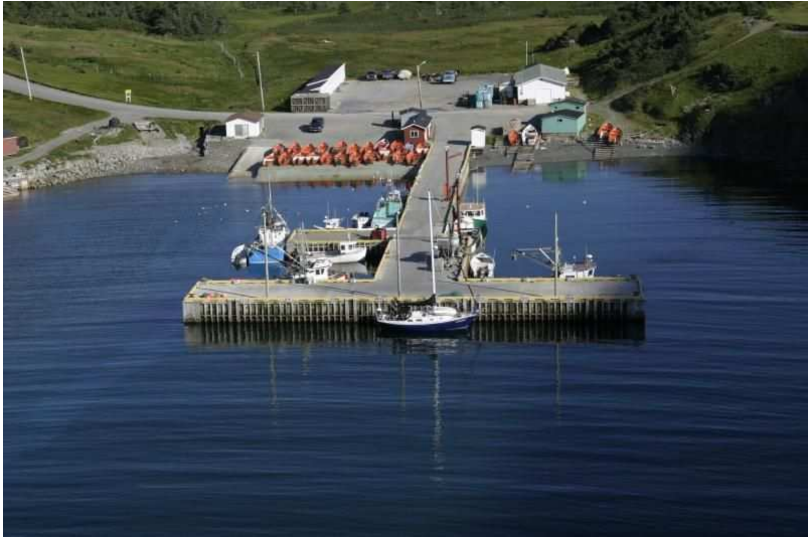
Site Photograph: Aerial view of Little Port dredging area.
