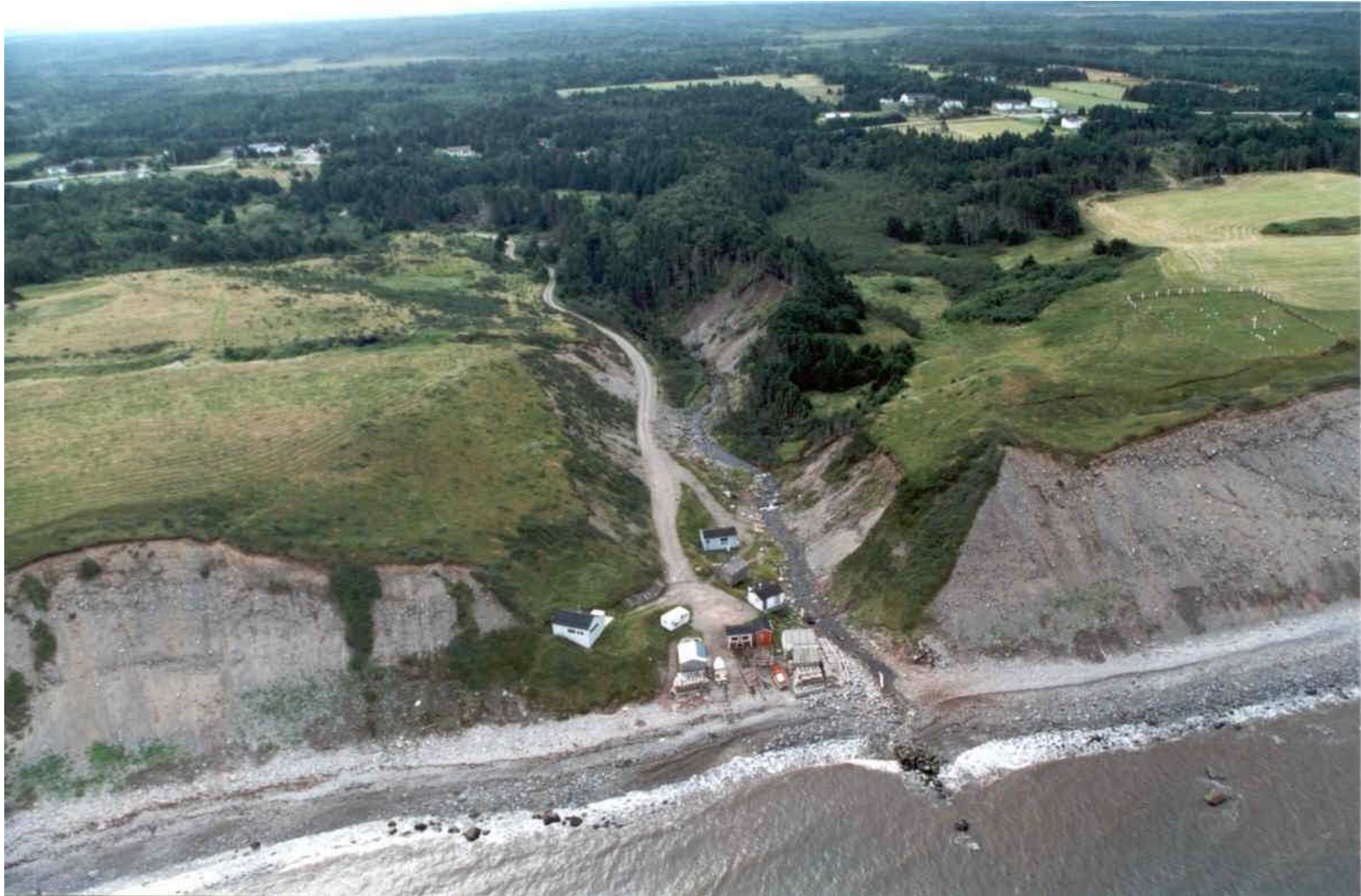
Site Photograph: Aerial View of Heatherton beach levelling site.
