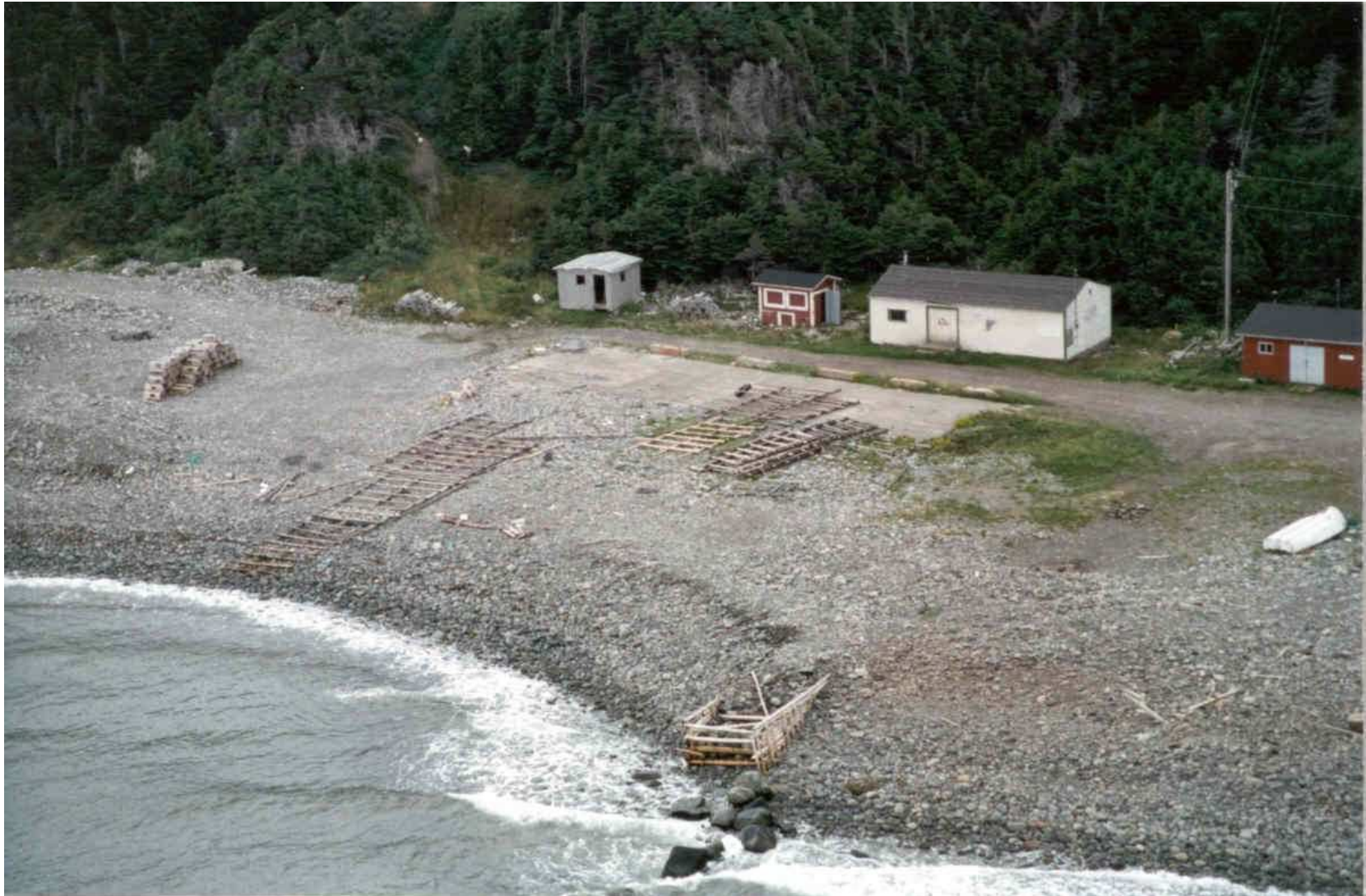
Site Photograph: Aerial View of Highlands beach levelling site.
