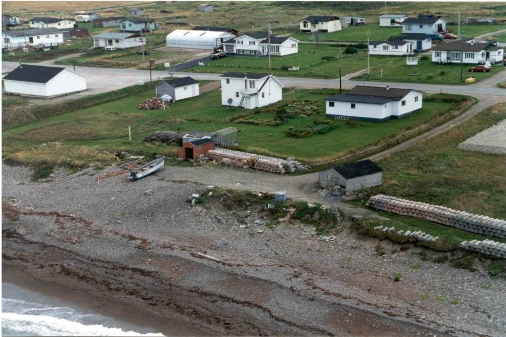
Site Photograph: Aerial View of Mainland beach – Moraze’s Landing beach levelling site.
