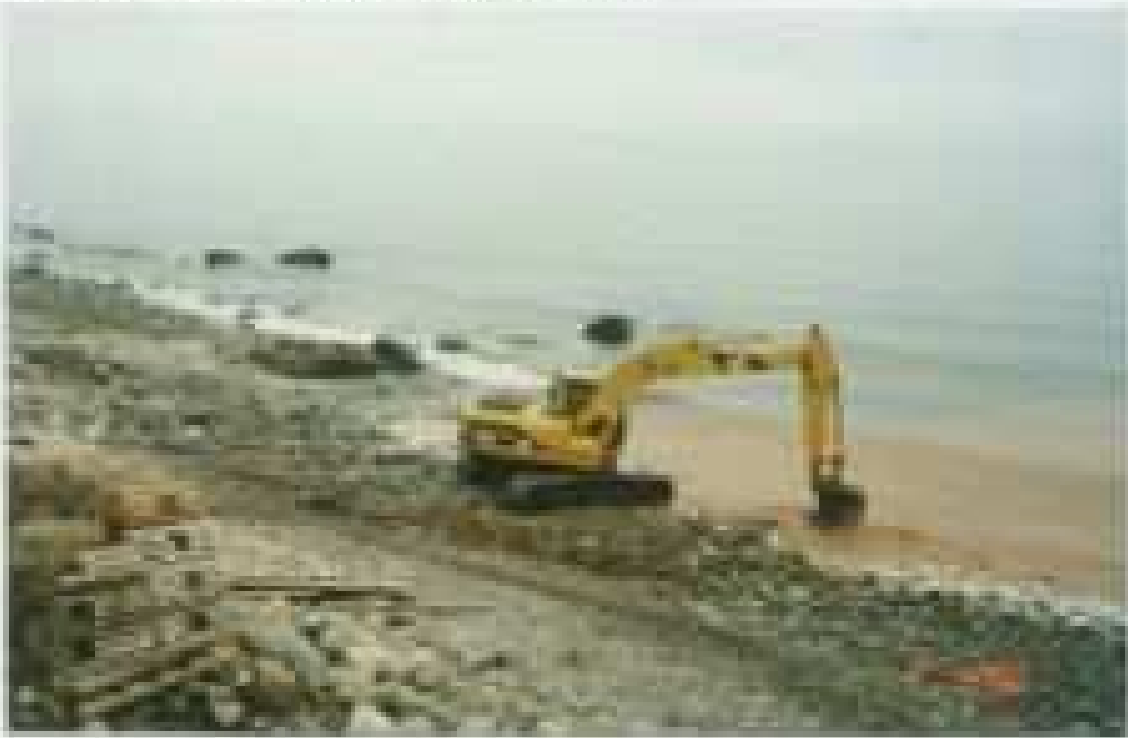
PHOTO 2 SEAL BROOK - DREDGING BASIN
