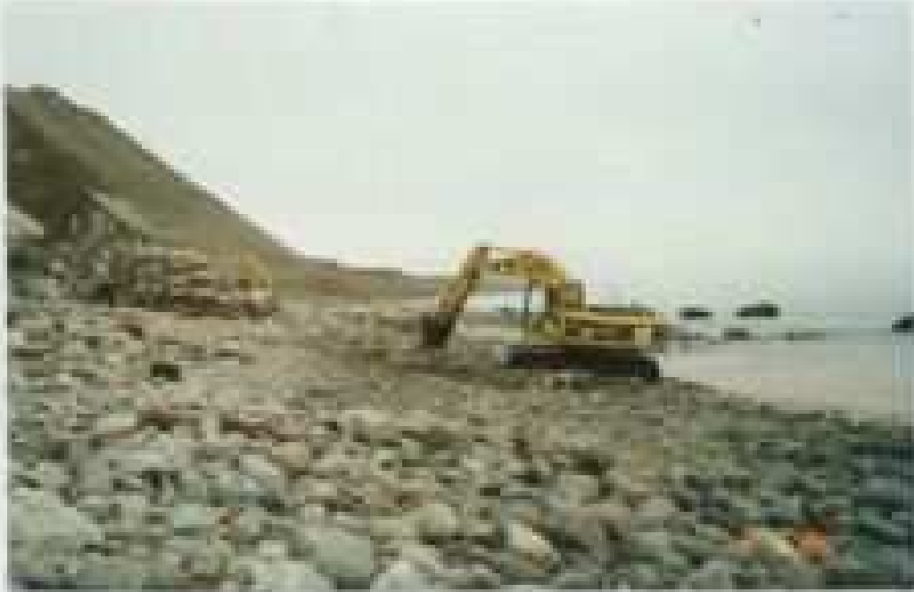
PHOTO 1 SEAL BROOK - BEACH GRADING
