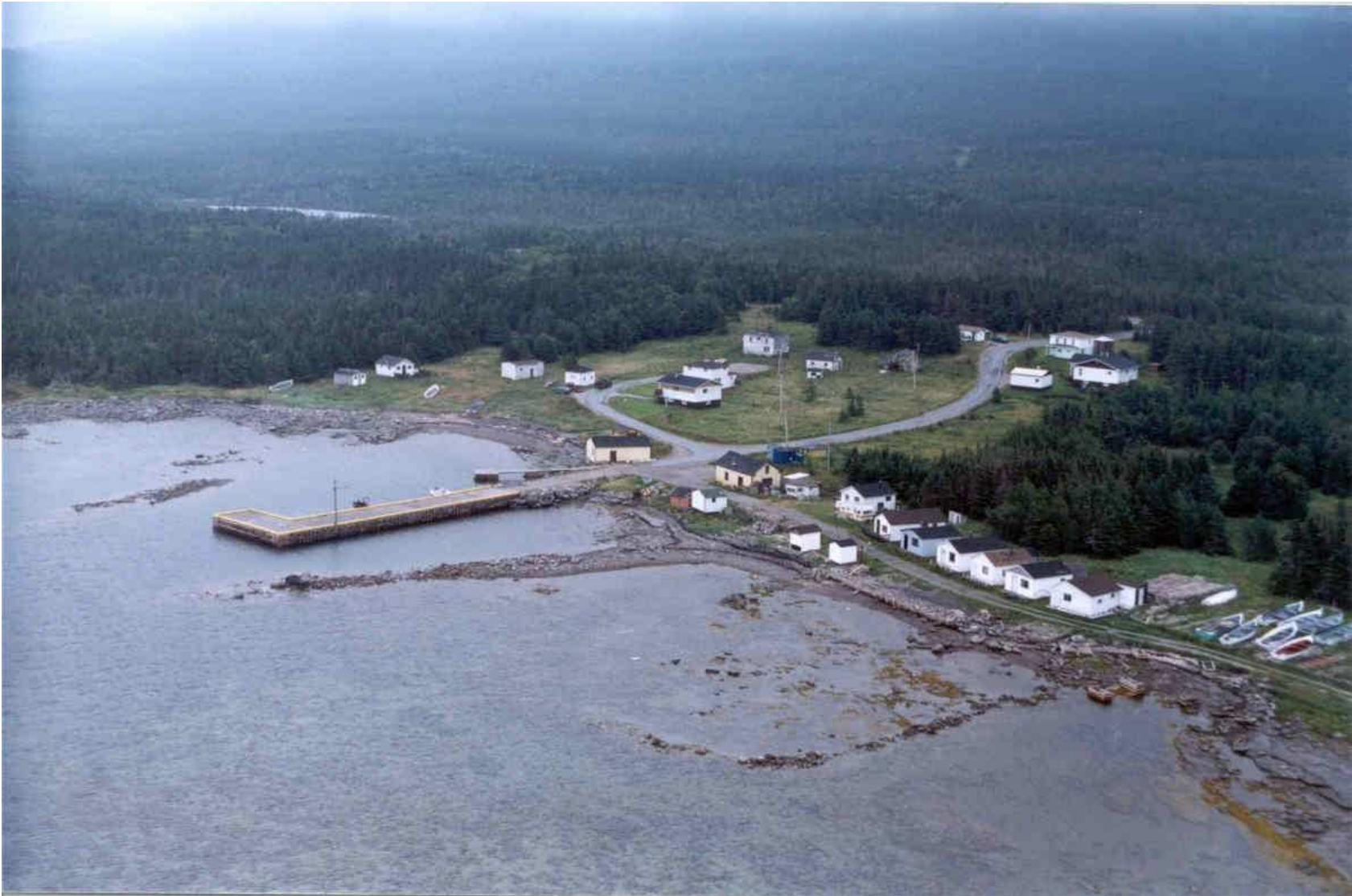
Site Photograph: Aerial View of Barr'd Harbour dredging site.
