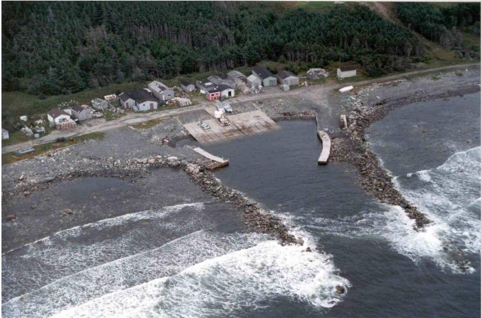
Site Photograph: Aerial View of Three Mile Rock dredging site.
