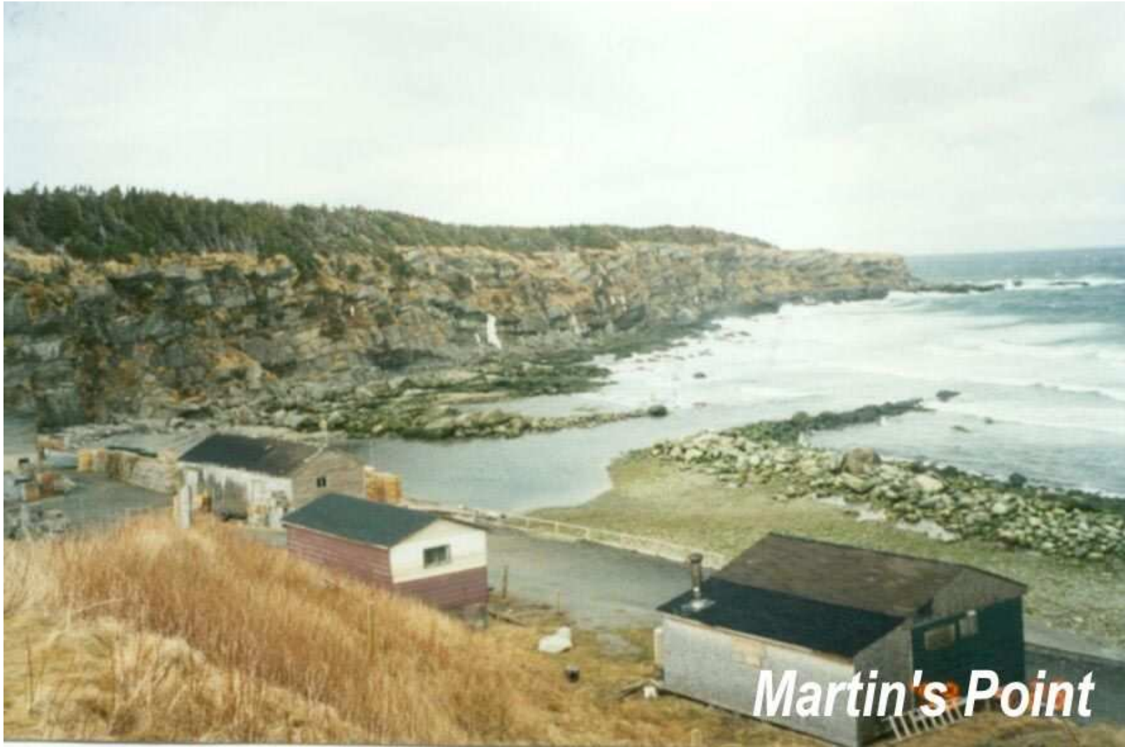
Site Photograph: Aerial View of Martin's Point dredging site.
