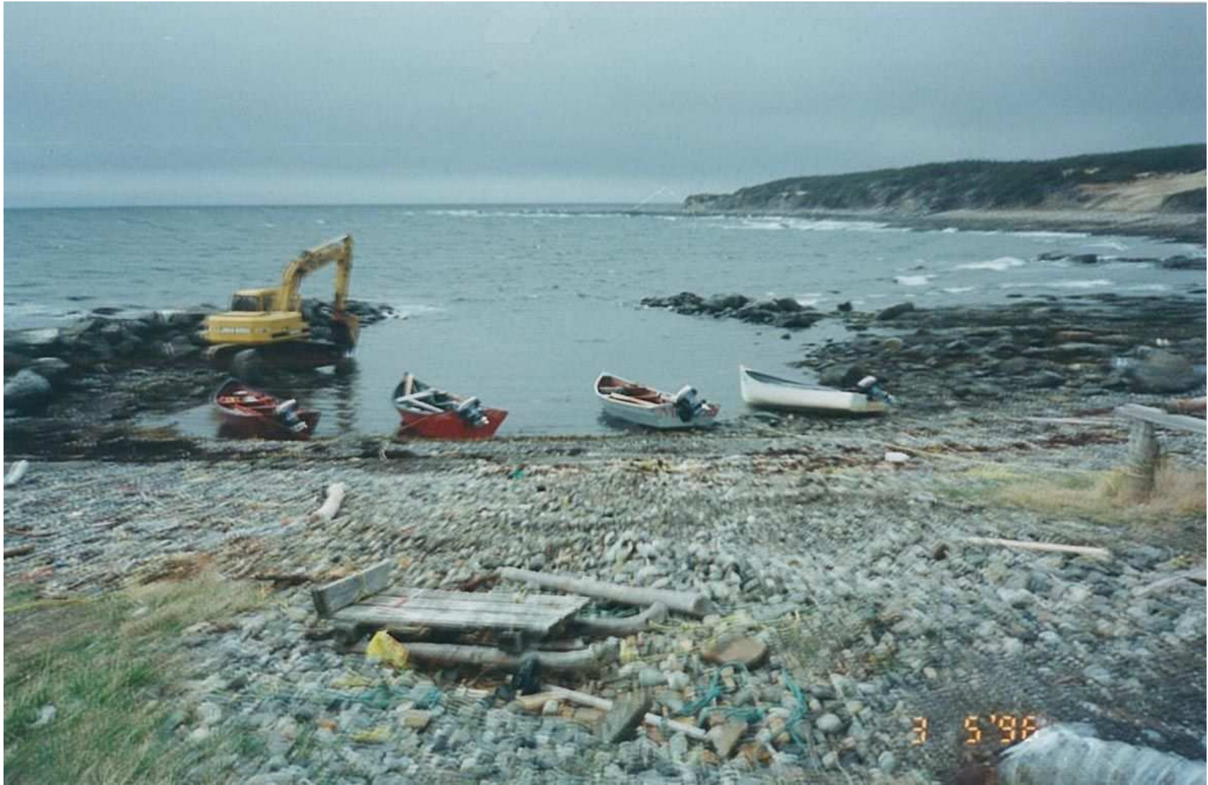
Site Photograph: Aerial View of Lobster Cove dredging site.
