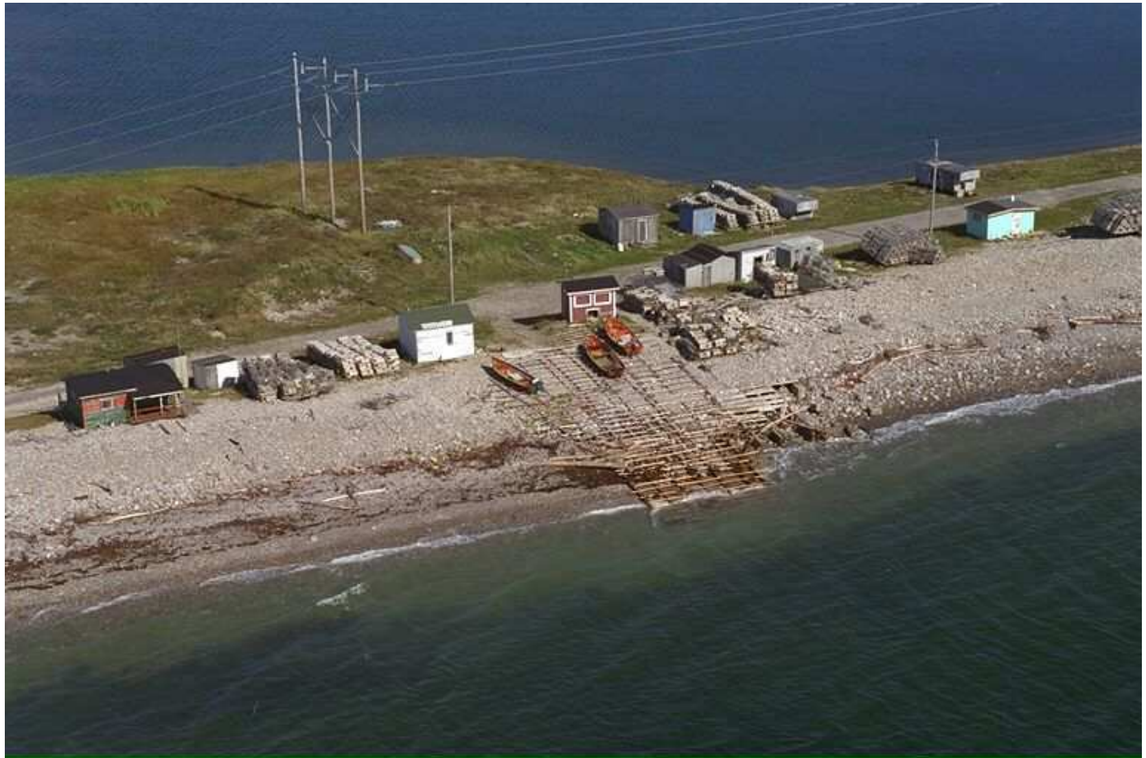
Site Photograph: Aerial View of Gravels dredging site.
