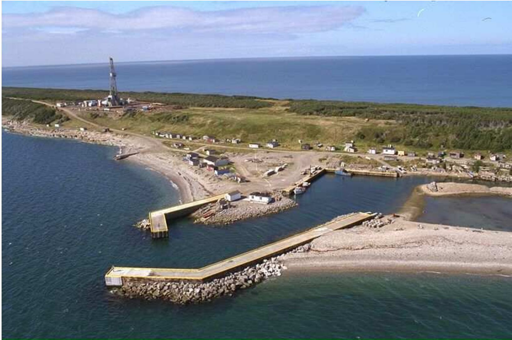
Site Photograph: Aerial View of Blue Beach dredging site.
