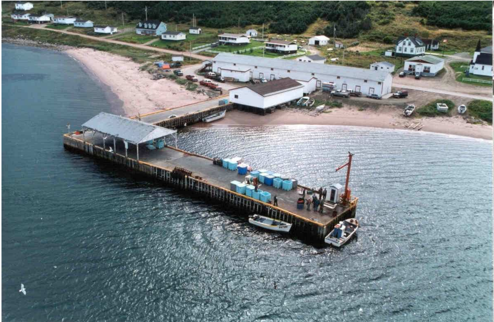
Site Photograph: Aerial View of Forteau Cove dredging site.
