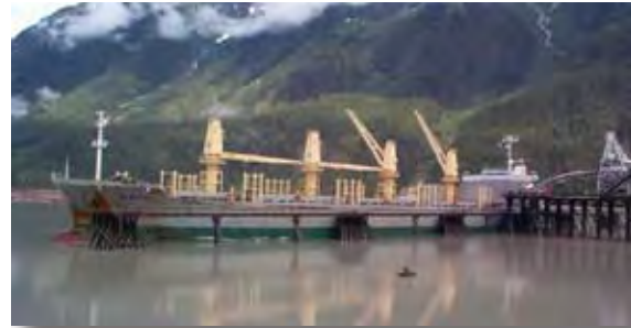
Stewart Bulk Terminal
