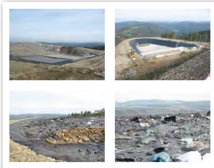
Figure 18: Final Oily Waste Disposal Solution for the Prestige Spill Oil Waste - a landfill
