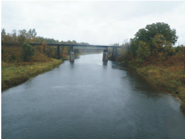
Lower Pinewood River: PIN-18 Facing Upstream
