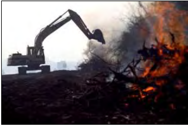
Credit: BC Hydro
