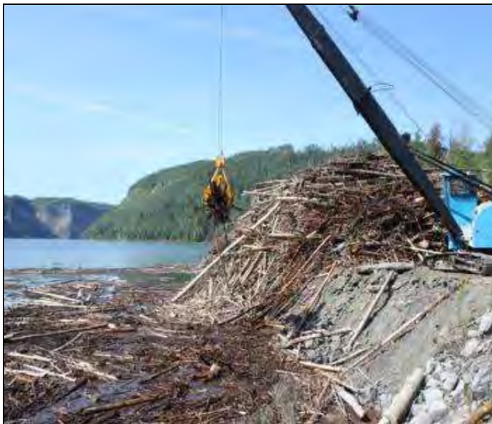
Photograph H-8 Grapple crane removing debris from Dinosaur reservoir trap
