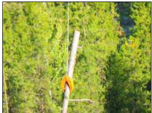
Credit: BC Hydro
