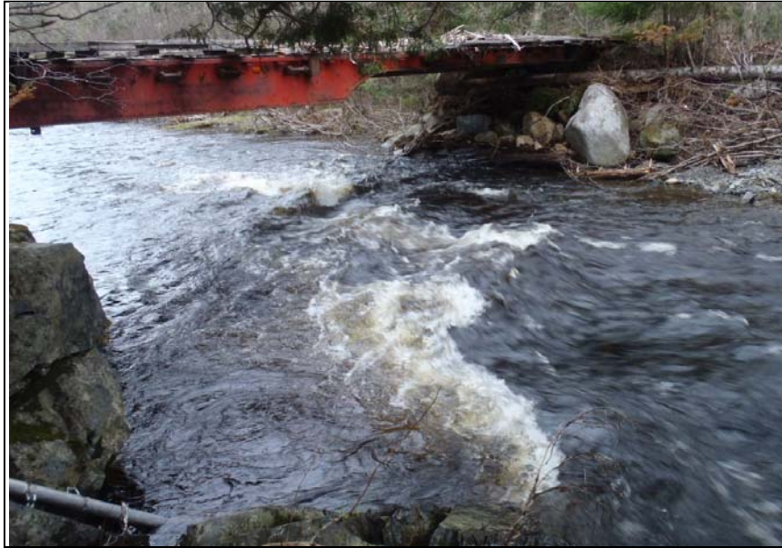
PHOTO 5 – Pressure Transducer Location at Station NB-2B
