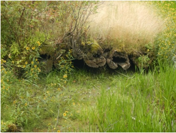
Figure 17: View west showing the log 'ramp' leading to the south bank of Dixie Creek, east of the forestry operations bridge.
