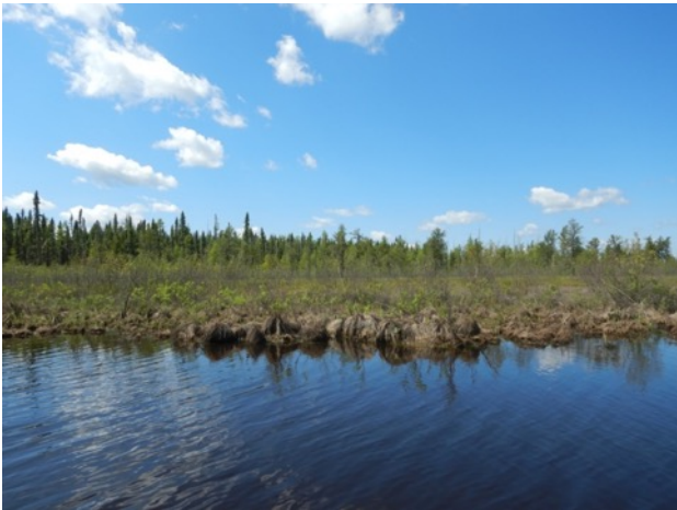
Figure 18: View south showing typical shore conditions on Dixie Creek upstream from the bridge. Note that the tufts of grass are in standing water.
