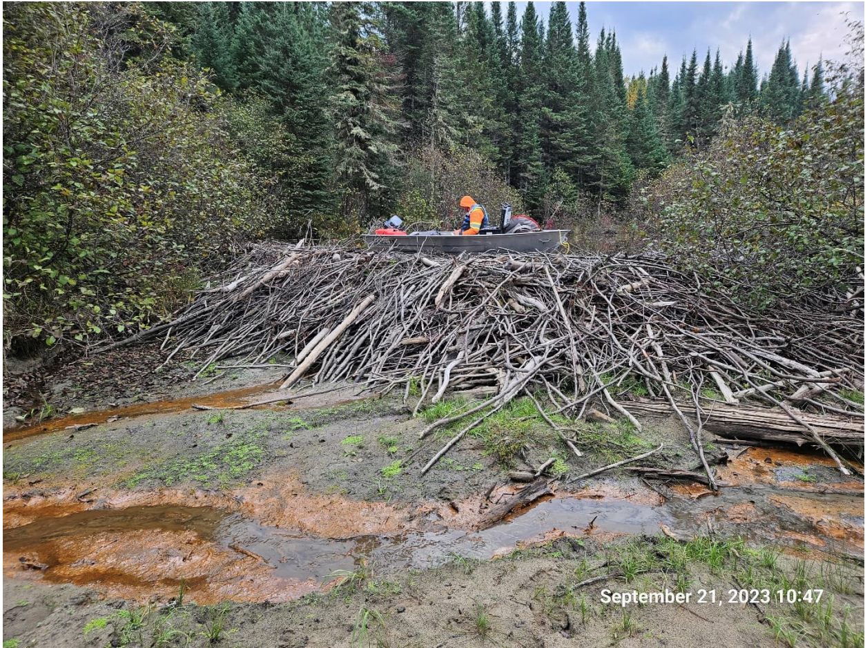
Figure 4.3: Photograph of beaver dam downstream from the Dixie Lake outlet (HF-07)
