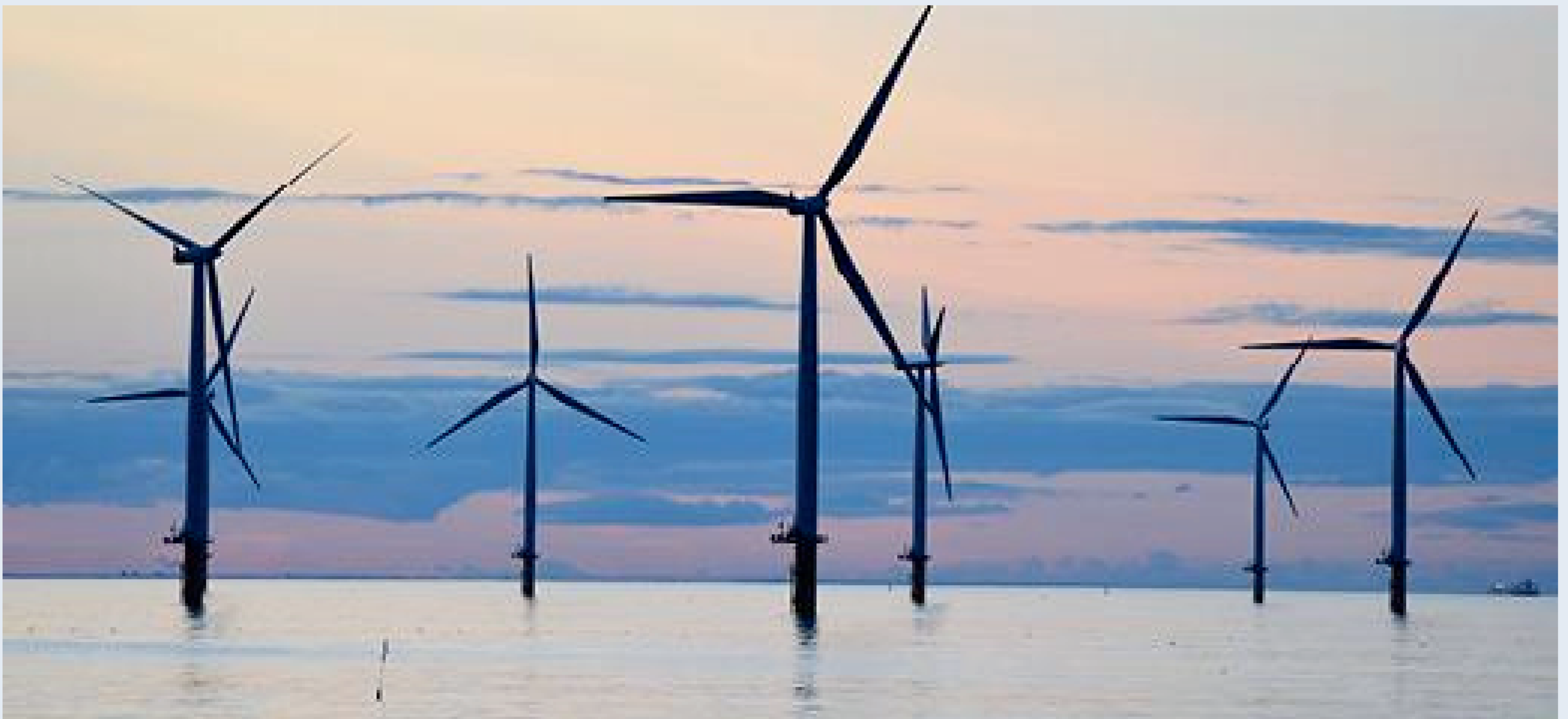
Galloper Offshore Wind Farm in the UK, Source: Green Investment Bank
