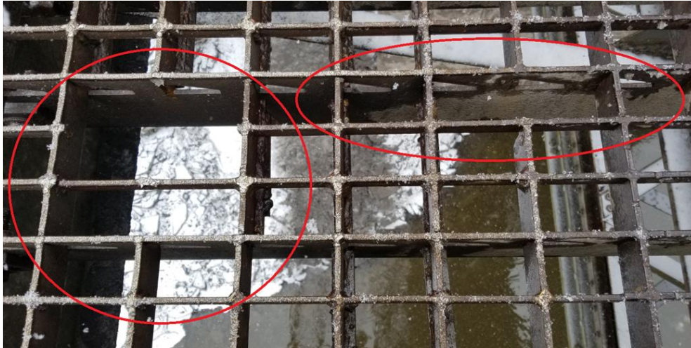
Figure 10-6: Local failure of the East lane grating
