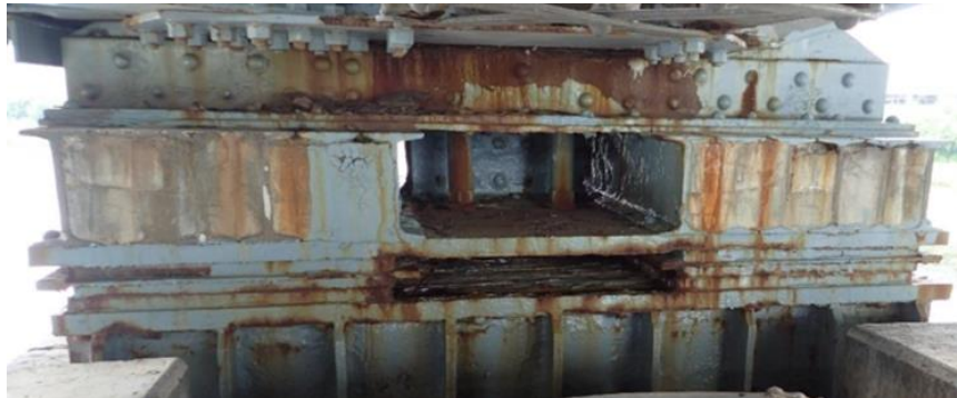
Figure 10-8: Bridge bearings
