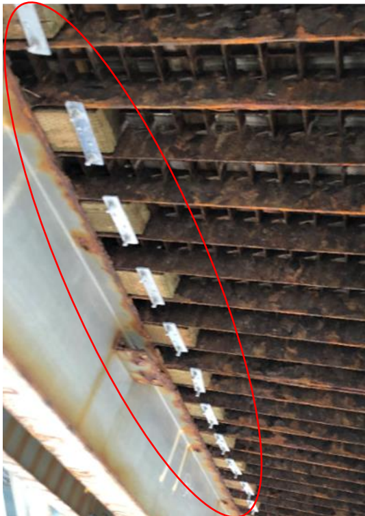
Figure 10-4: Timber wedges to provide short term support to the grating.
