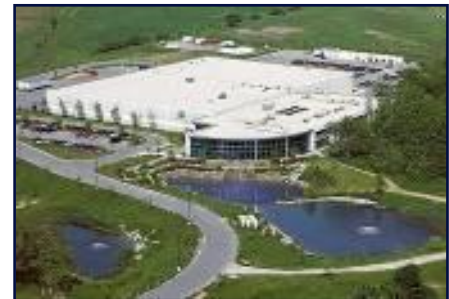
SUEZ’s global UF/MBR center of excellence located in Oakville, Ontario, Canada
