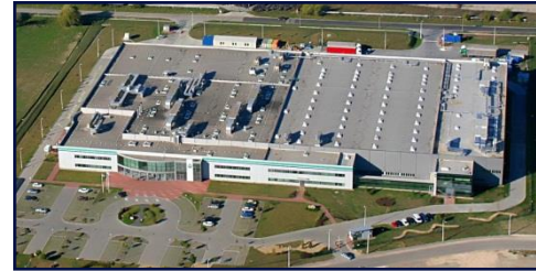
membrane manufacturing plant located in Oroszlány, Hungary
