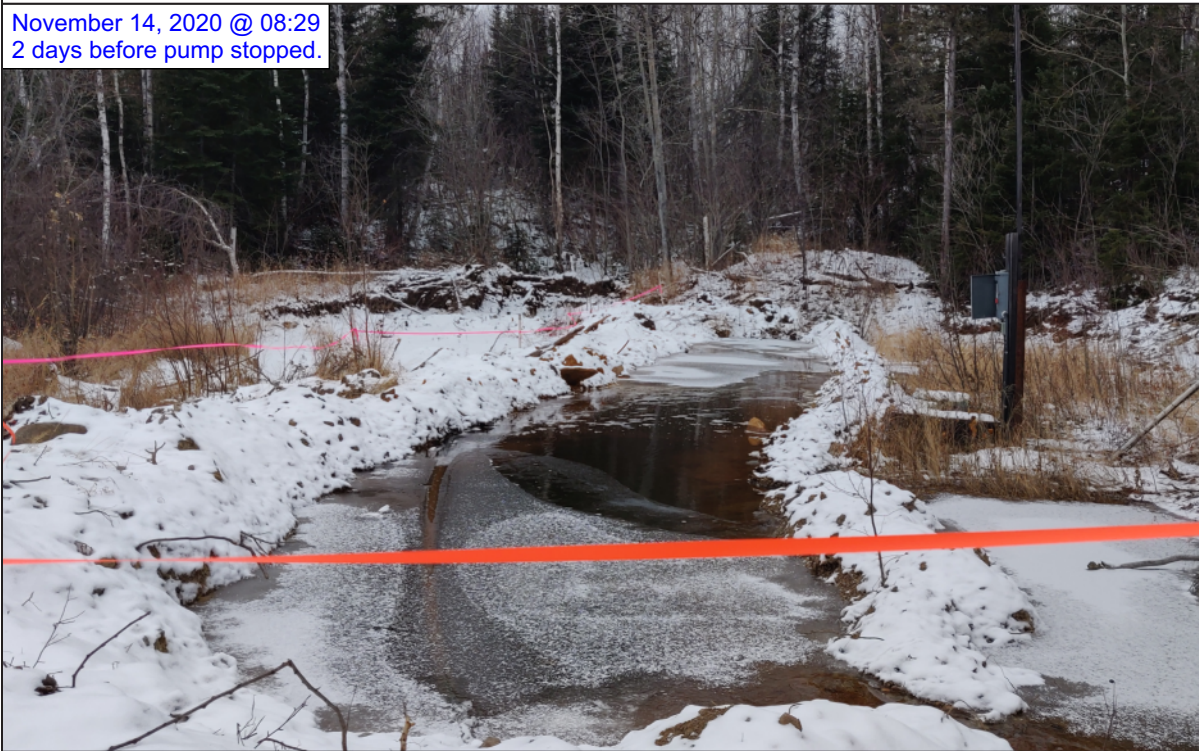
Figure 6.3 Photographs of soak-away trench for long-term aquifer test discharge from Test Well (SPW20-001).
