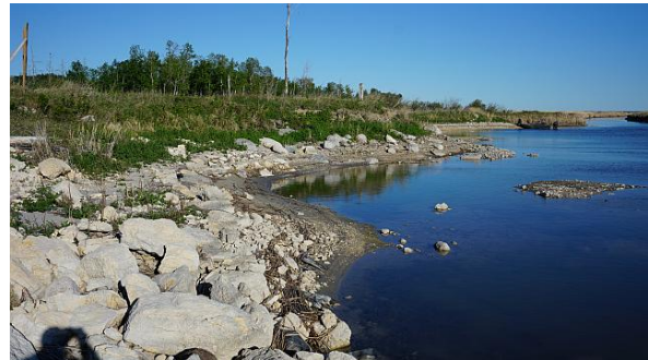
B: Minor Sand Accumulation East of the Cut-off Berm
