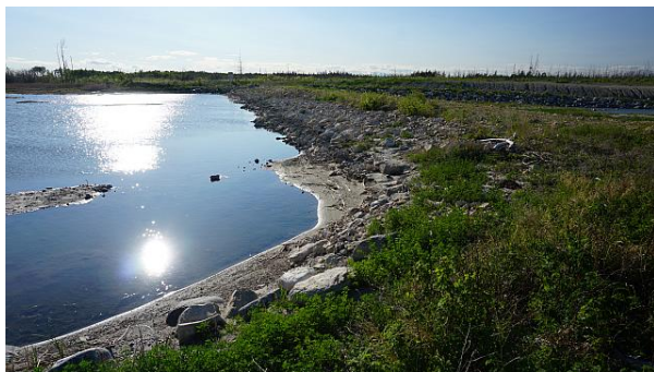
C: Lake Side of Cut-off Berm and Small Sand Deposit at the Waterline
