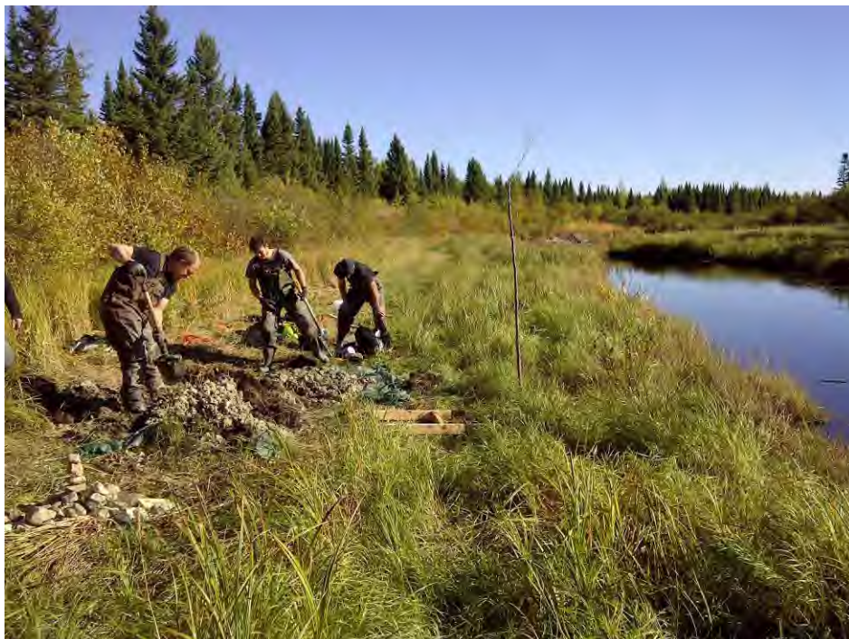
Photo 6 – Backfilling testpit
