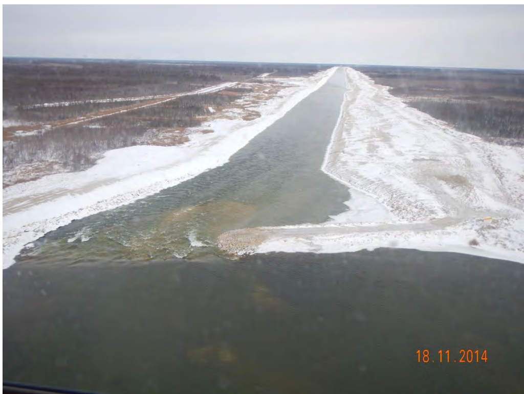
Photo 2. Reach 1 Inlet, looking downstream.
