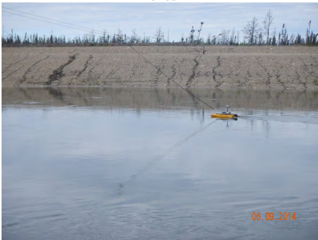
Photo 1. Reach 1 Cableway, South Shore
