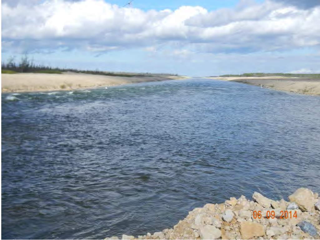
Photo 5: Reach 1 Inlet, looking downstream.
