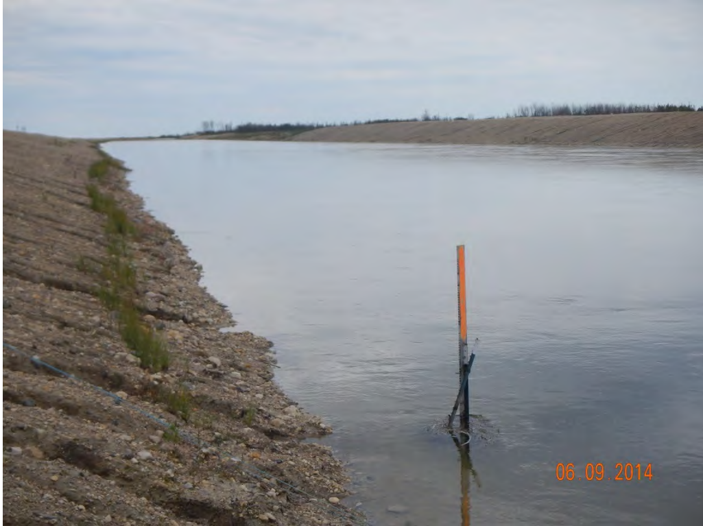
Photo 3: Reach 1 Cableway, South Shore looking upstream.
