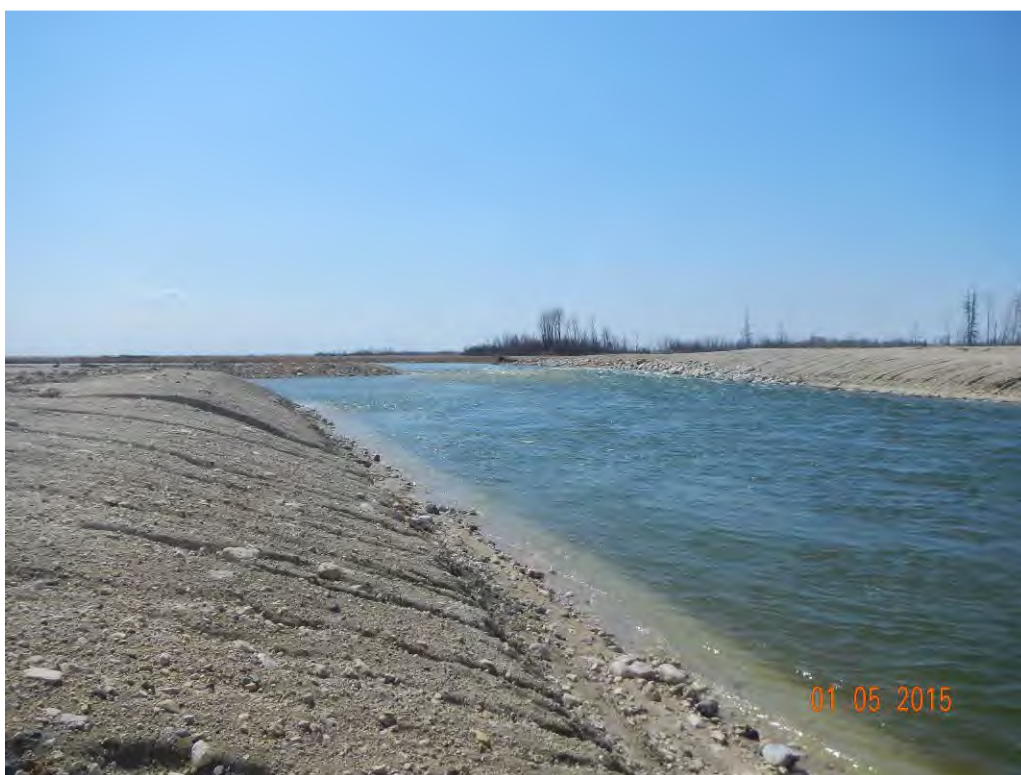
Photo 10. Bench Mark R1-I-A looking west, U/S
