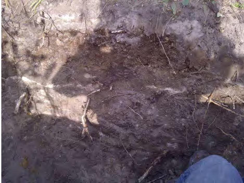
Photo 1 – Side wall of testpit
