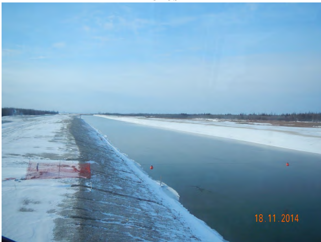
Photo 1. Reach 1 Cableway, South Shore, looking upstream.
