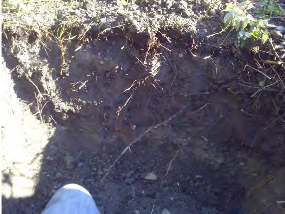
Photo 1 – Side wall of testpit
