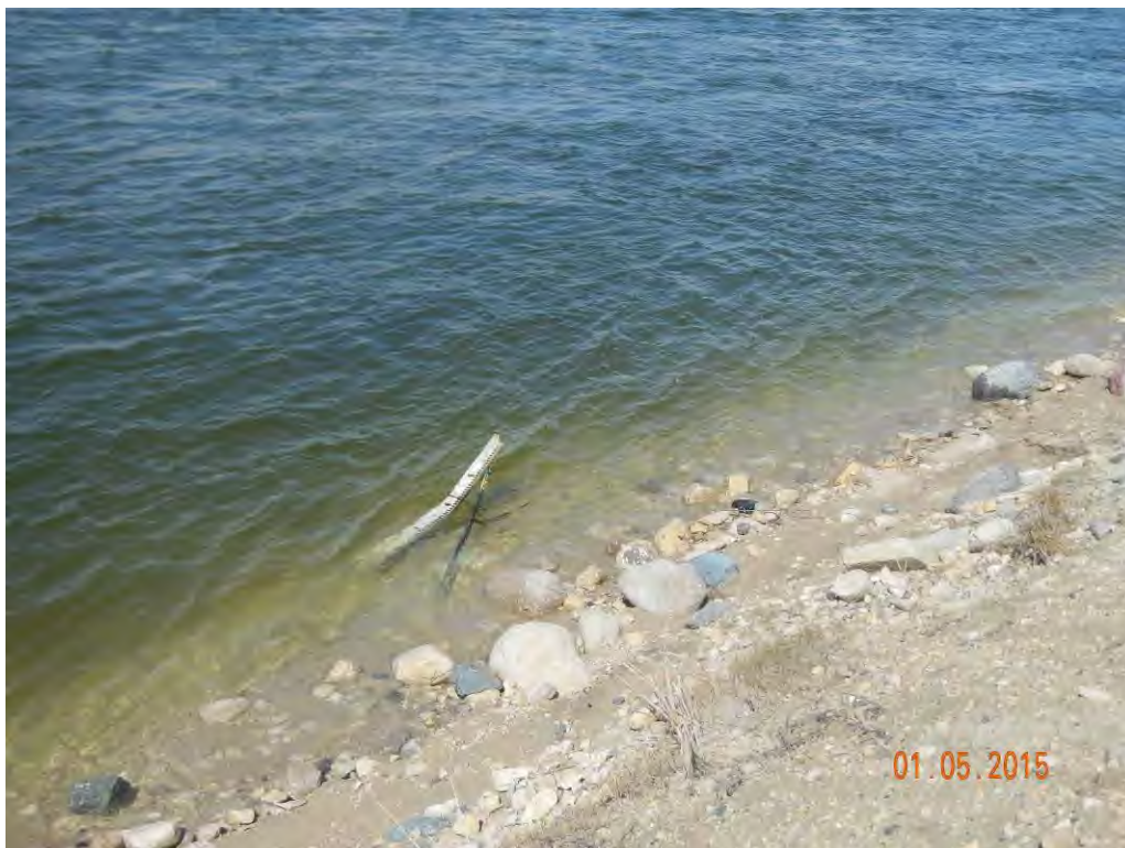
Photo 11. At Bench Mark R1-I-A, damaged gauge board
