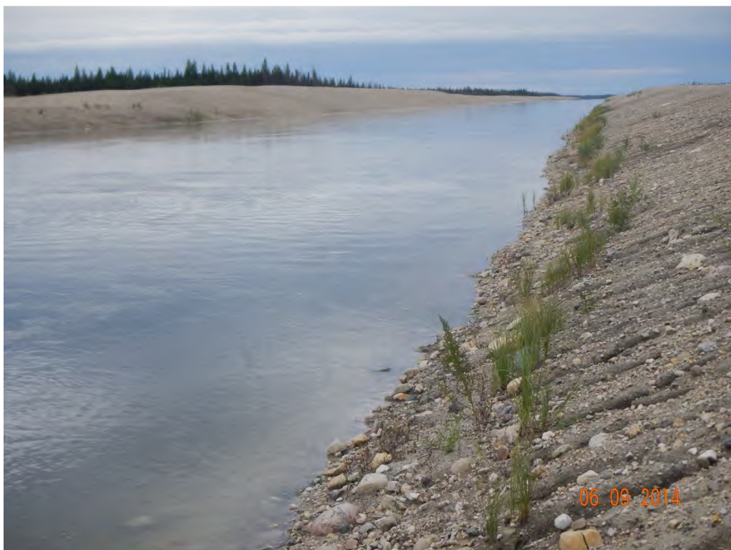
Photo 2. Reach 1 Cableway, South Shore looking downstream.
