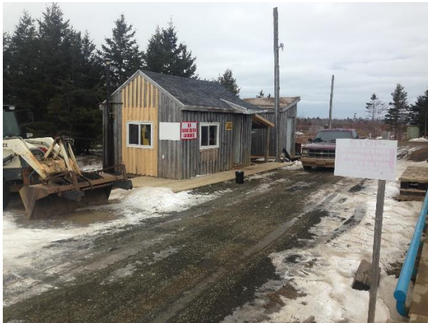
Photo 18: On site office and scale house.
