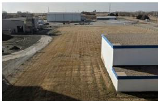
Capped mound of Hallam facility
