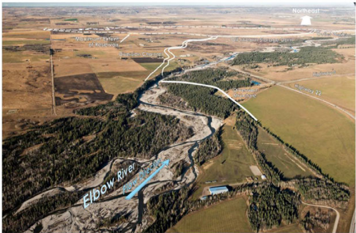
Figure 3-4 Looking Northeast towards Diversion Structure, Diversion Channel, Off-stream Storage Reservoir and Off-stream Storage Dam Locations
