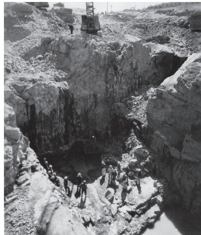
Bedrock excavated during the construction of NPD
