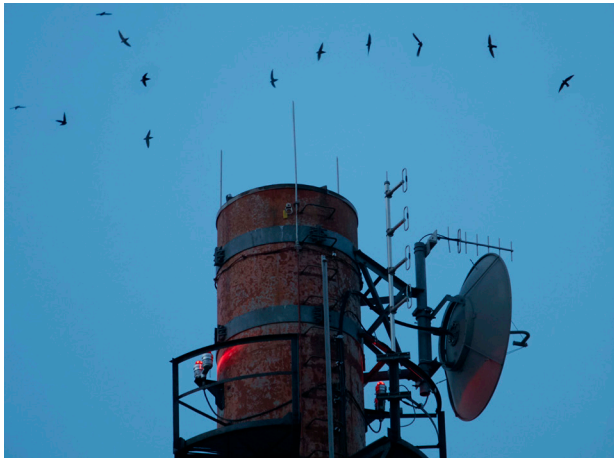
Chimney swifts entering the NPD ventilation stack at sunset
