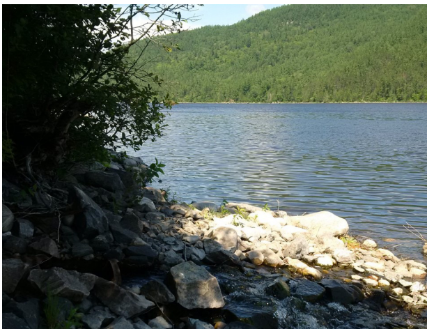
A view from the NPD site; for more than 50 years, NPD has been safely operated and maintained beside the Ottawa River
