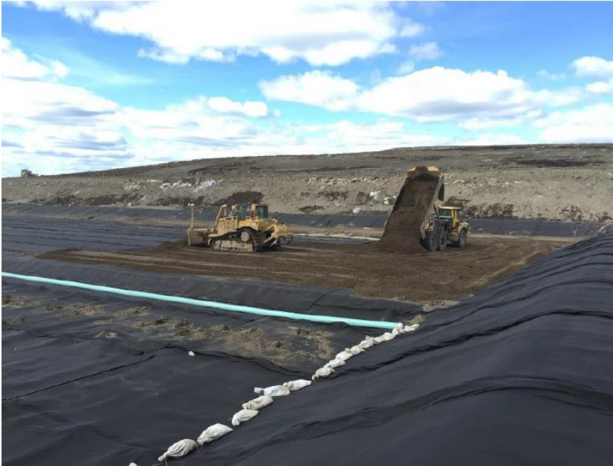
Photograph 2-1: Typical Cell Construction Photo
