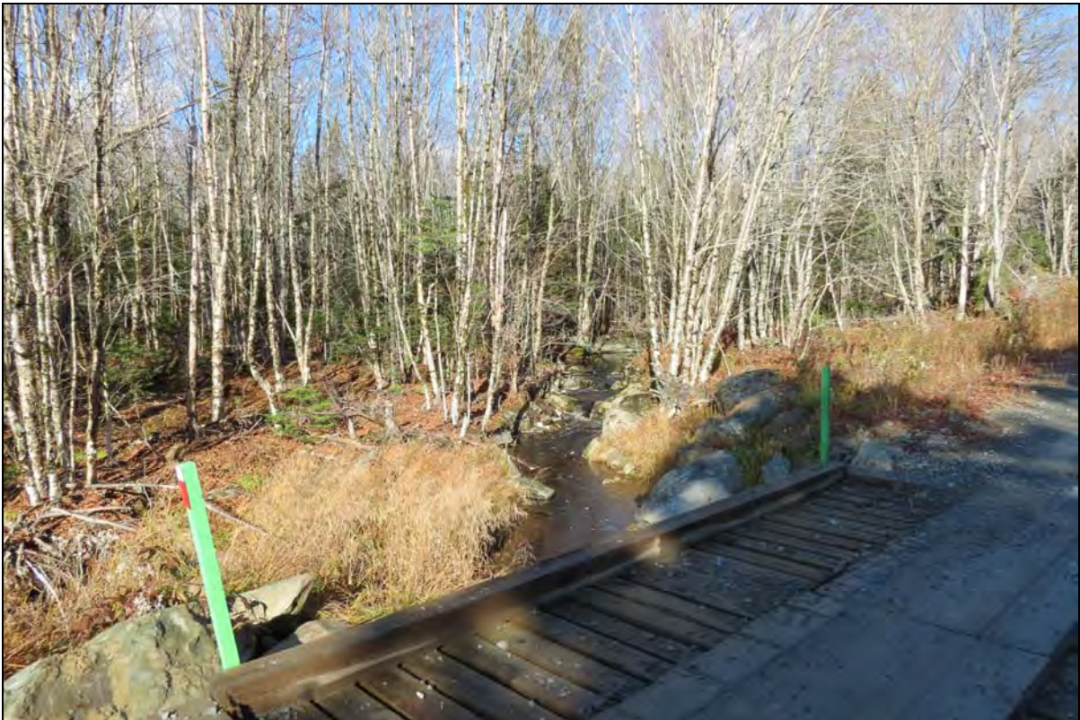
PLATE 1: Small water crossing in the haul road study area; facing southwest. November 13, 2015.
