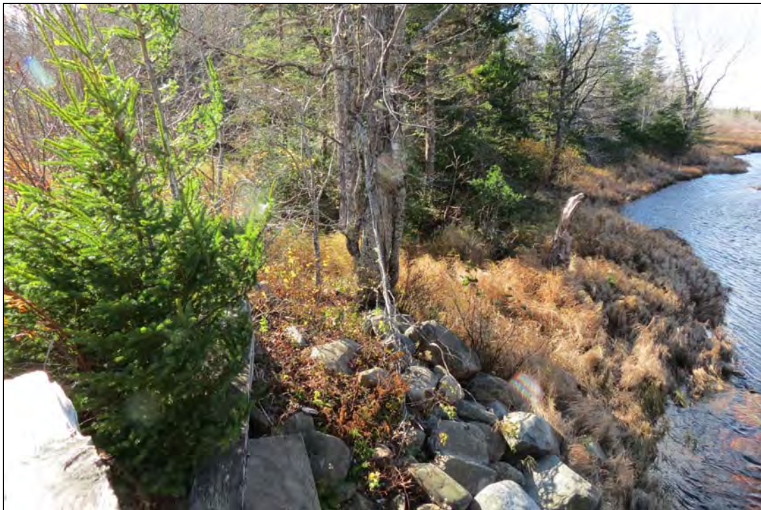
Plate 8: Morgan River crossing; facing west. November 13, 2015.
