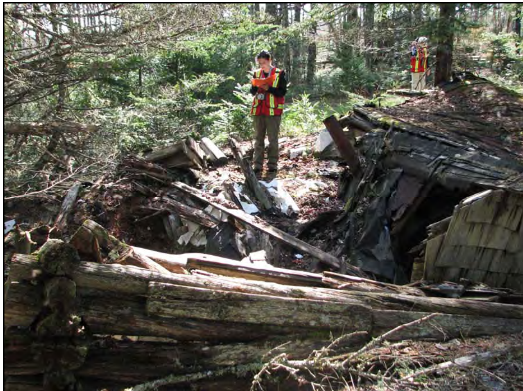
PLATE 7: Site 1: Remains of collapsed wooden structure; facing southwest.
