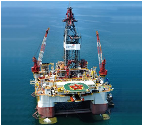
Figure 12. Seadrill West Sirius semi-submersible platform.
