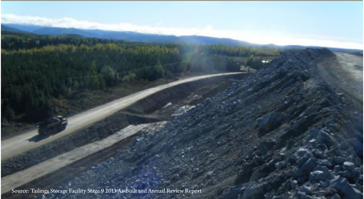
Exhibit 21: Perimeter Embankment slope with area stripped for buttress, submitted by the EOR to MEM in March, 2014
