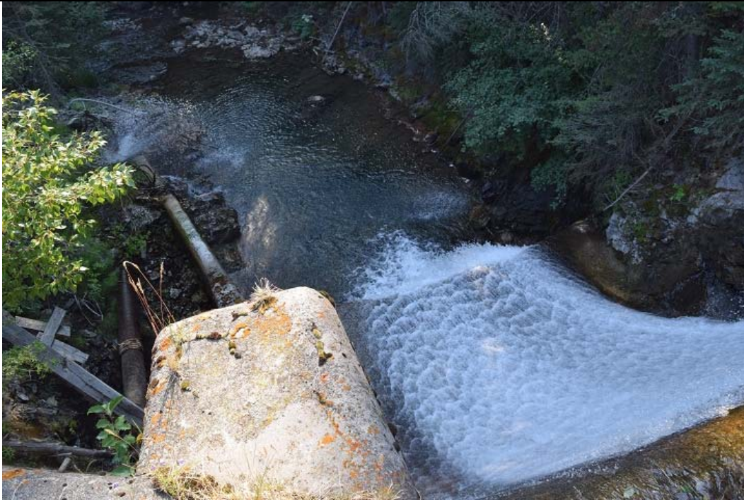
Photo 3 – Drop Structure and Water Release From Dam
