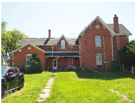
Plate 9: East facade, looking west
