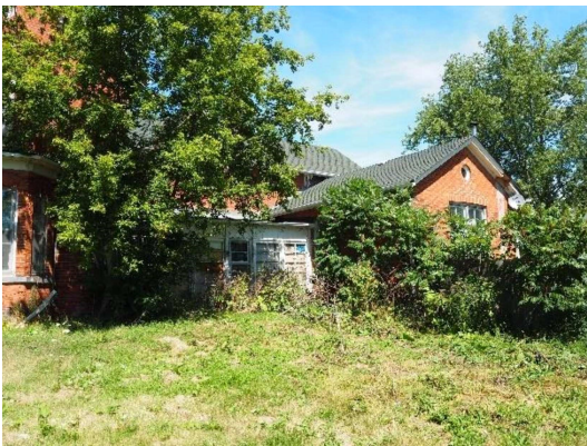
Plate 4: East façade, looking west
