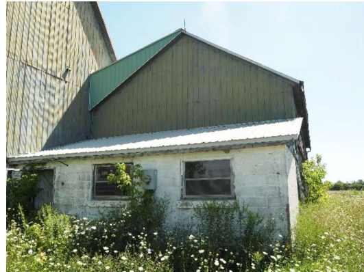
Plate 25: Concrete block addition on south façade, looking east
