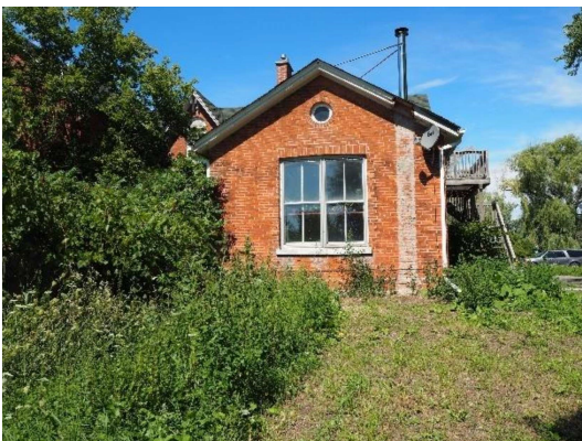
Plate 6: One storey portion of the east façade, facing west
