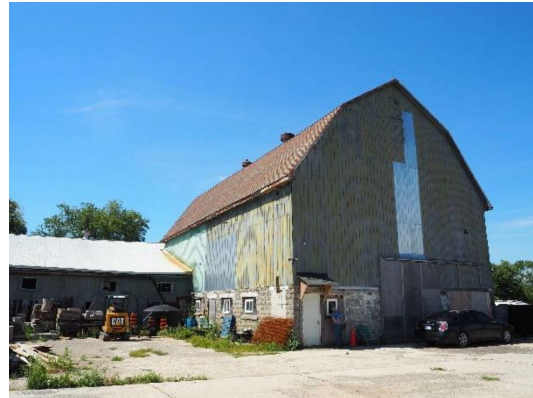
Plate 19: North and east façades showing gambrel roof and metal cladding, looking south
