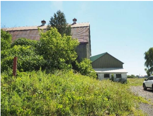
Plate 26: West façade, looking east
