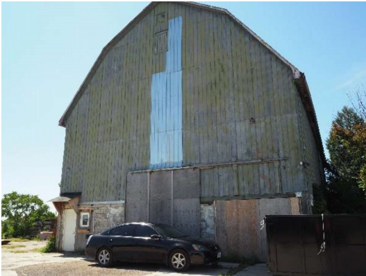
Plate 18: North façade, looking south
