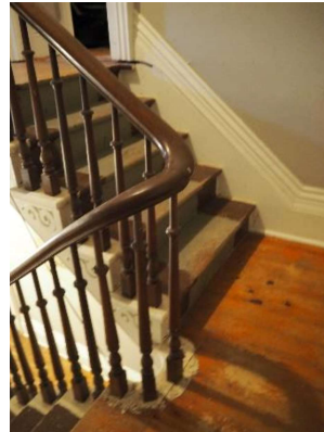
Plate 11: Grand central staircase's carved newel post, also shows original pine floors and trim
