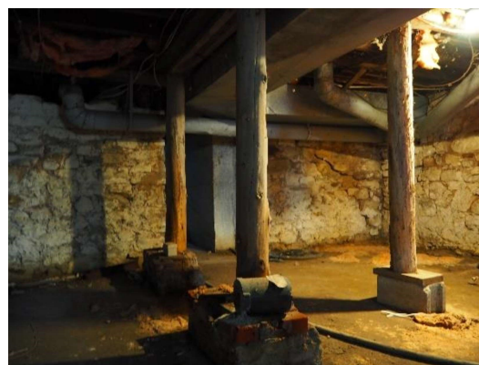
Plate 17: Timber support posts
