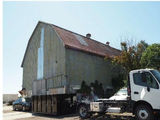
Plate 27: west façade, looking southeast
