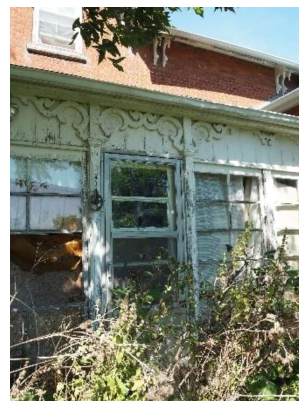
Plate 5: Covered porch on east façade, looking west
