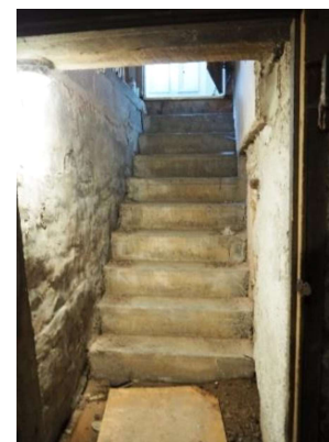
Plate 15: Concrete staircase which provides basement access
