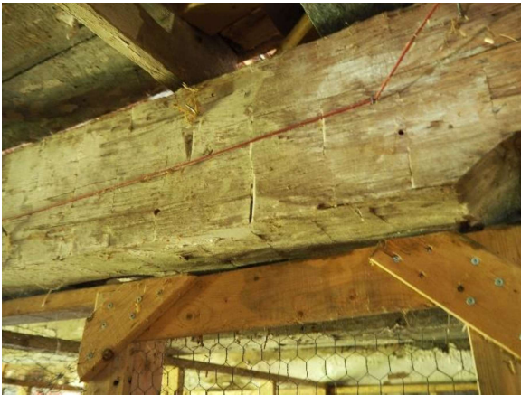
Plate 43: Hand hewn interior beams showing little damage
