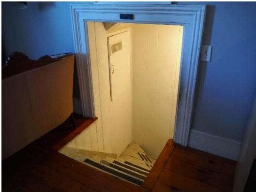
Plate 12: "Service" style back staircase descending view, also showing original pine floor and trim
