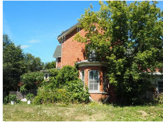
Plate 3: East façade, looking west
