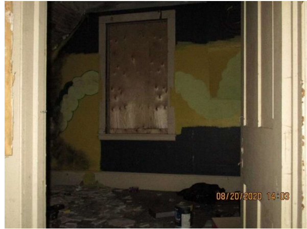
Plate 13: Interior upstairs room
