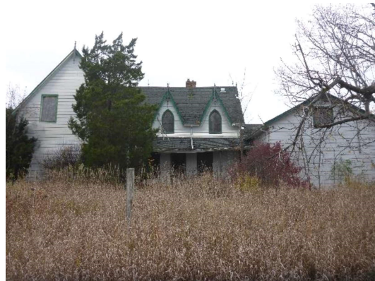
Plate 9: East façade, facing west
