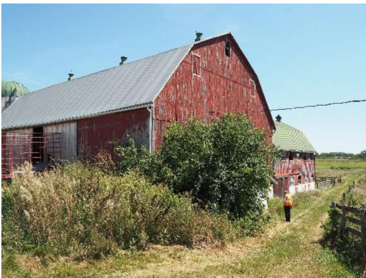
Plate 18: West and south facades, showing bank incline, looking northeast
