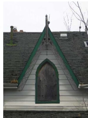
Plate 11: Arched window, bargeboard, and finial on east façade, facing west
