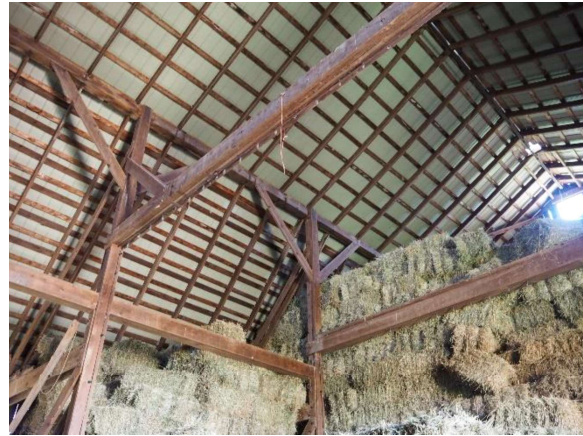
Plate 26: Machine cut beams, posts, and joists
