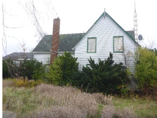
Plate 5: West façade, looking east
