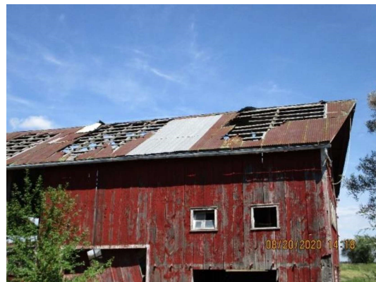
Plate 43: Gable roof section of the barn
