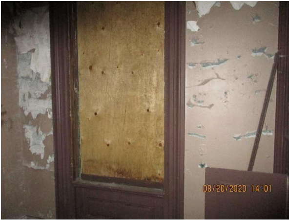
Plate 12: Interior window with plywood covering
