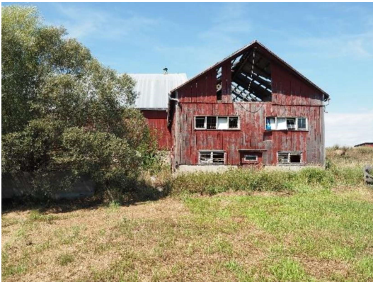
Plate 24: East façade of gable roof rear addition, looking west
