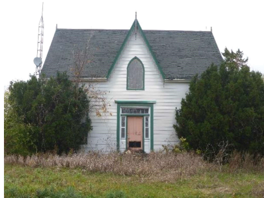
Plate 3: South (front) façade, looking north
