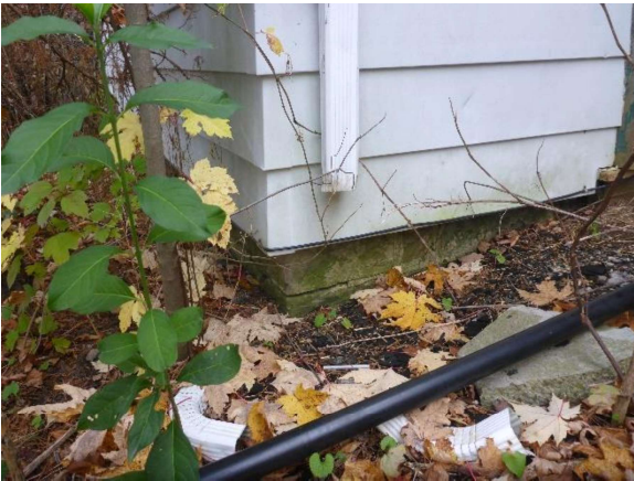
Plate 30: Downspouts draining to foundation
