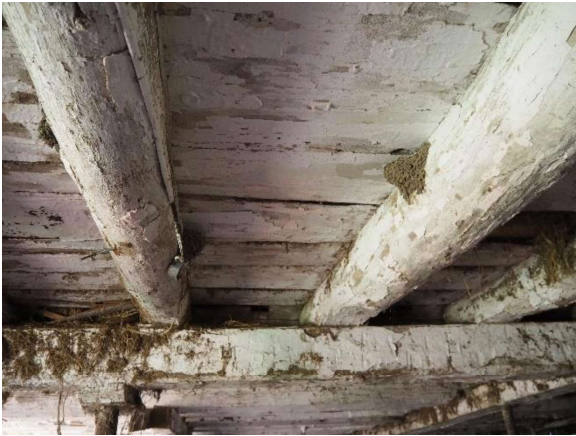
Plate 25: Hand hewn beams
