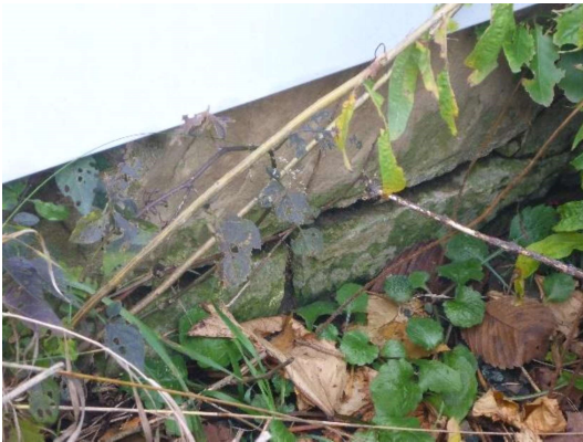
Plate 4: Cut stone foundation on the south façade, looking north
