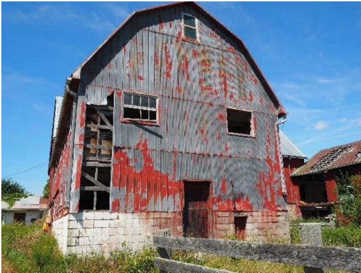
Plate 22: East façade of rear gambrel roof addition, looking west
