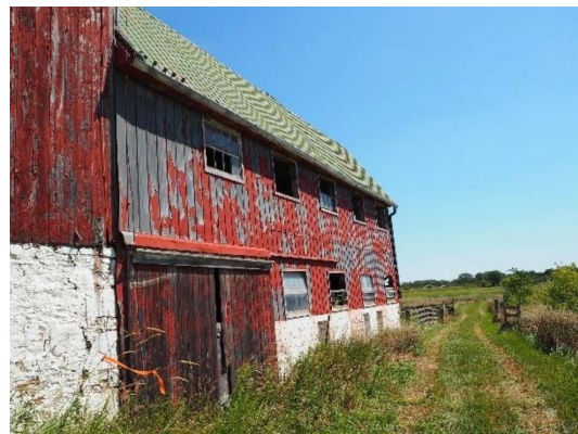
Plate 21: South façade of rear gambrel roof addition, looking northeast
