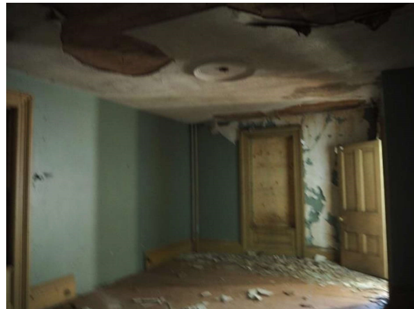
Plate 15: Interior front living area
