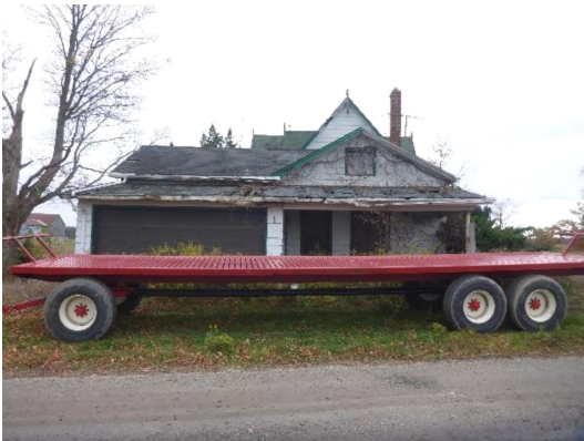
Plate 8: North façade, facing south
