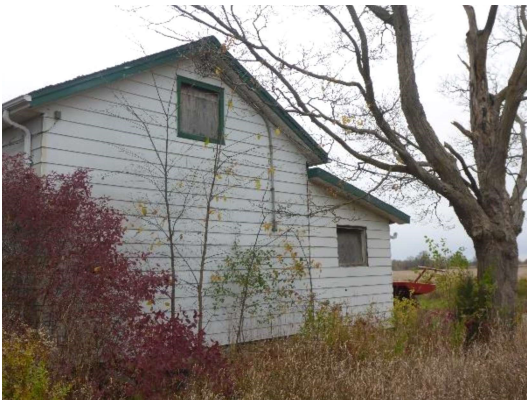
Plate 10: Garage, east façade, facing northwest
