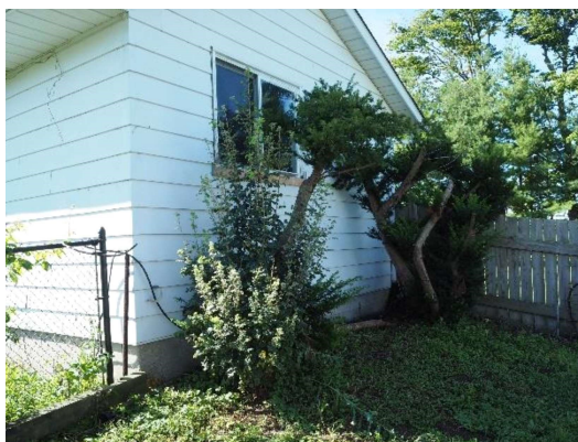
Plate 11: Northwest façade of gable roof addition, looking south
