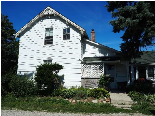
Plate 6: Southeast façade, looking northwest
