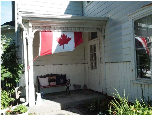
Plate 4: Front entrance and covered porch with decorative trim, southwest façade, looking north
