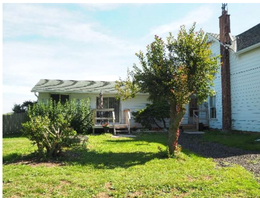
Plate 9: Southwest façade of gable roof addition attached to northwest side of residence, looking northeast
