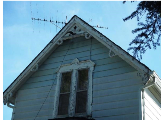
Plate 3: Bargeboard and decorative wooden window surround, southwest façade, looking north
