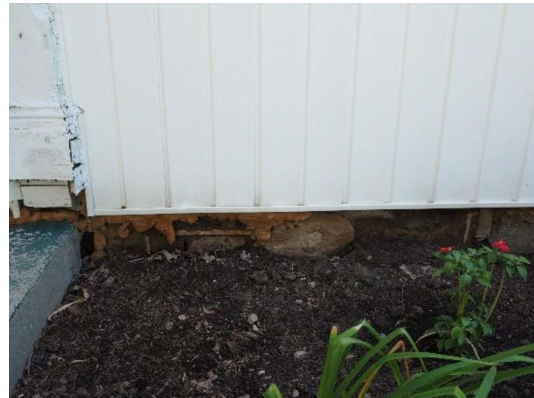
Plate 5: Stone foundation on southwest façade, looking northeast
