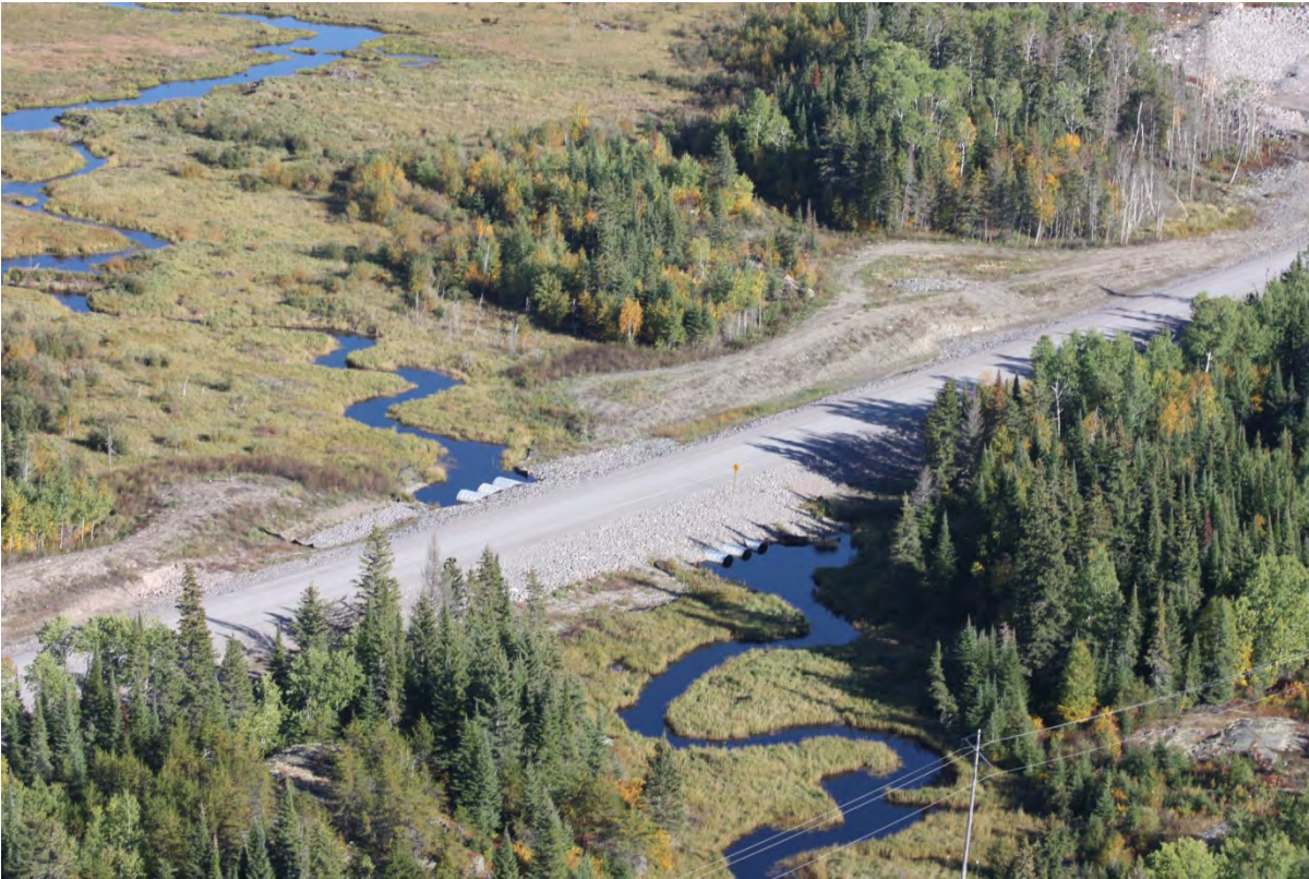
Photo 12: Stream Crossing – Three culverts (representative from P1)
