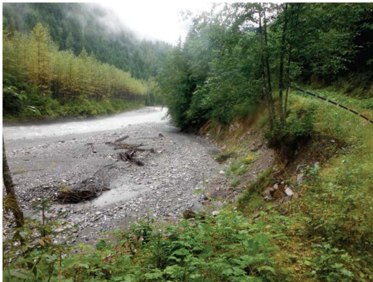
Figure 6-4: Lateral erosion and washout near station 15+000. Dashed line shows previous access road.
