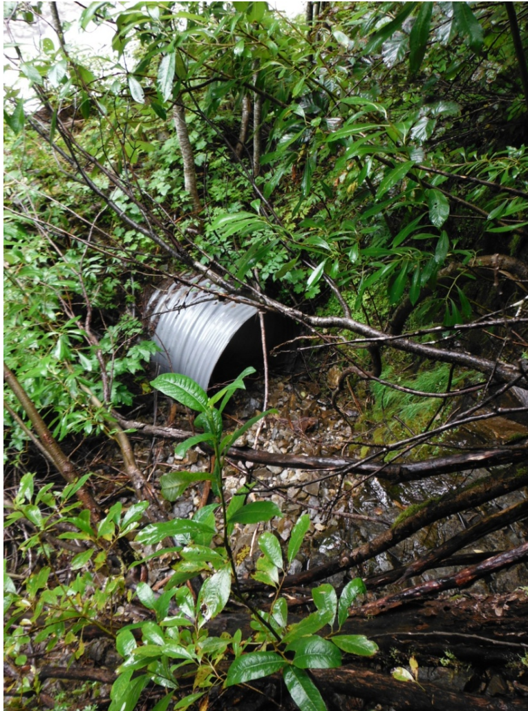
Figure 7-2: Culvert outlet below former road at Unnamed Creek 2.
