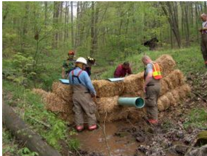
Figure 7-2. Photo depicting a rudimentary siphon dam.
