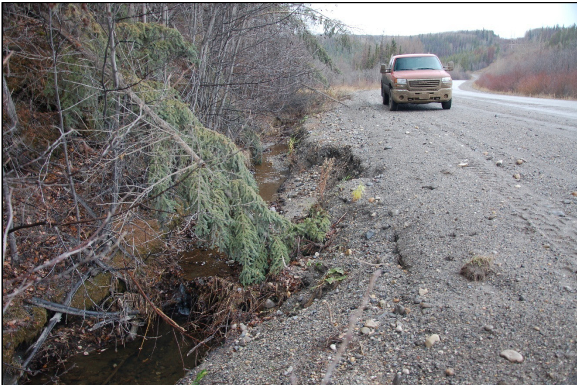
Plate 6. Wetland outflow through Murray FSR ditch between wetland complex and Murray River. – Nov 02, 2011.
