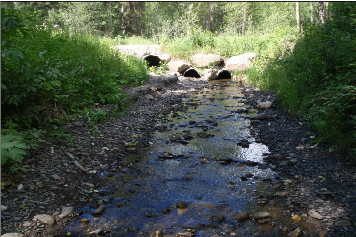
Twenty Creek – Reach 1; view upstream to Murray FSR culvert crossing (Aug 05, 2011).
