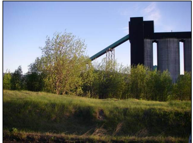
d) grass/short shrub (maintained) habitat near existing mine infrastructure (Transect MR06)
