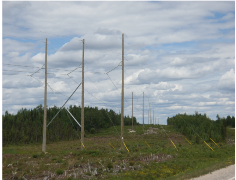
Photograph 4-1: Typical 230 kV Transmission Line and Poles
