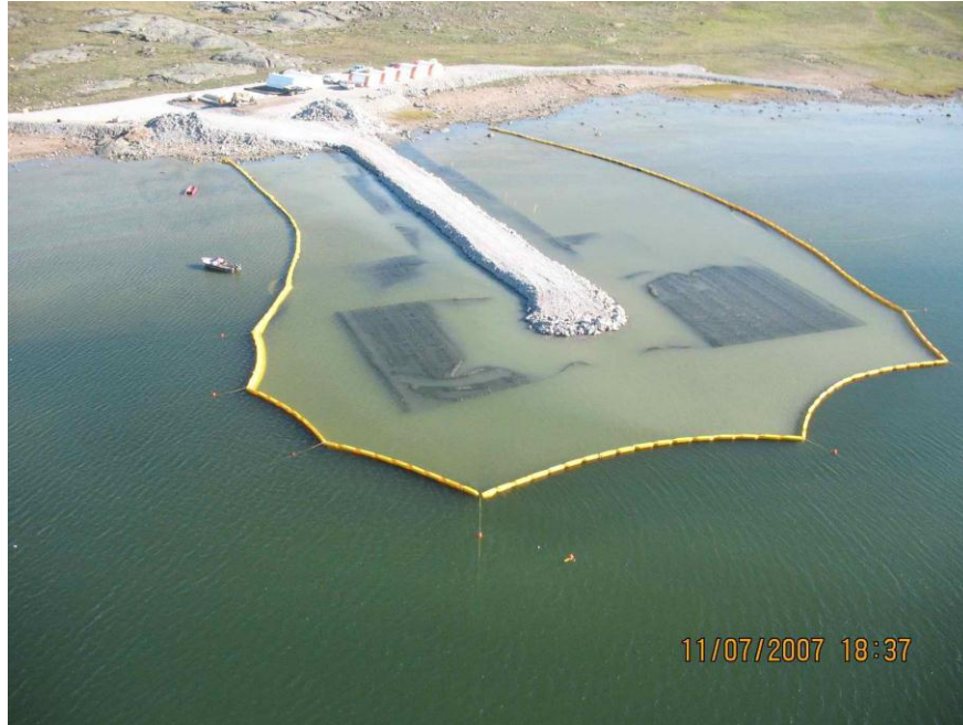
Photo 4. Silt curtain employed in a lake for waste rock deposition. Photograph courtesy of Pretium.
