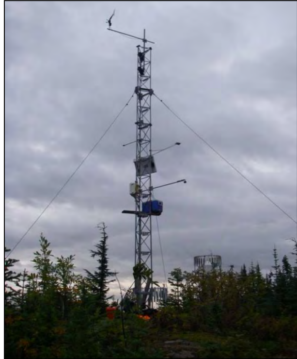
Plate 6.1-3. Wildfire Creek meteorological monitoring station, September 2012.
