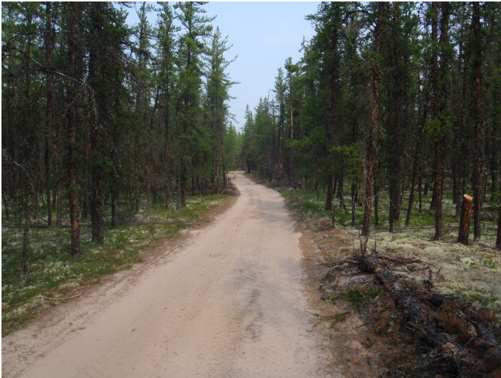
Photo 3.3-18: Assessed portion of road approximately 2.5 km south of Middle Lake
