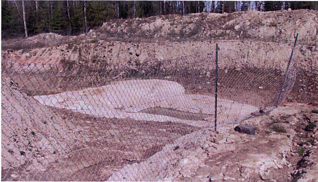
Image 17. View north above Beaver Dam of exploratory location and clay covered bedrock.
