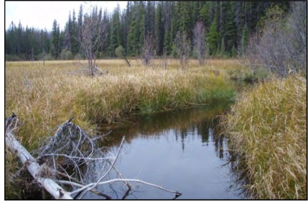
Plate 20. Big Bend Ck. TL-025 Transmission line crossing, fallen log and vegetation growth, October 2, 2012.
