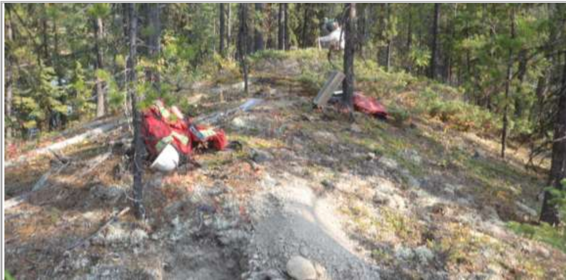
Photo 1.7-8: View Northeast at Crew Excavating Transmission Line Subsurface Test Location MF5
