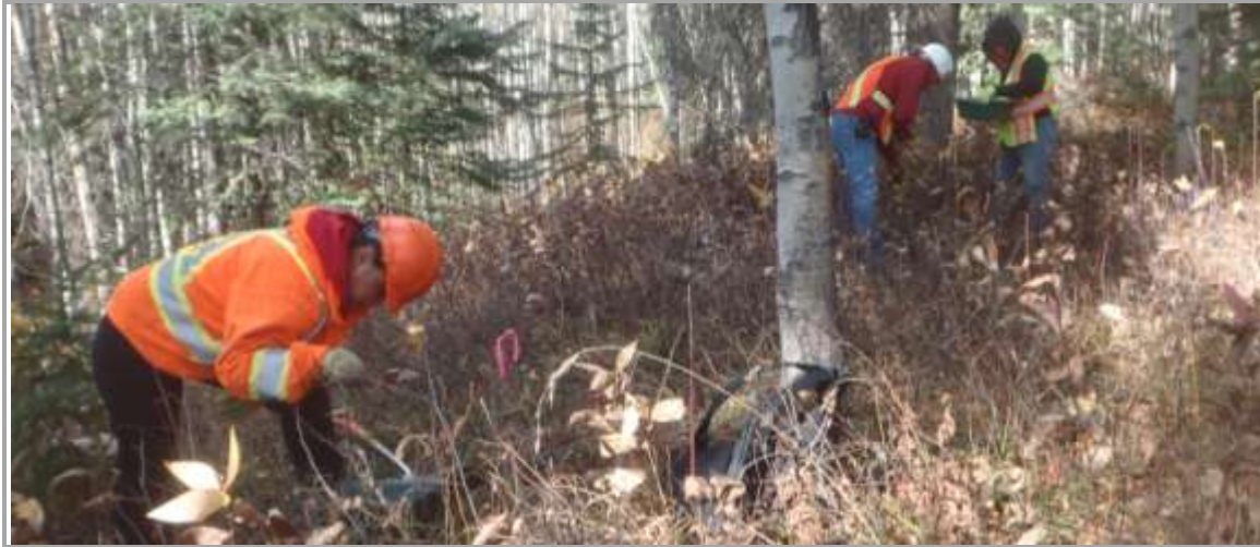
Photo 1.7-9: View West at Crew Excavating Transmission Line Subsurface Test Location NP3
