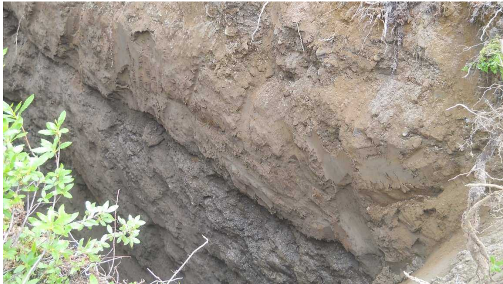
Photo 1: Thin groundwater seepage window at 3-4 ft bgs in excavation pit (Test Pit 9), July 8, 2013.
