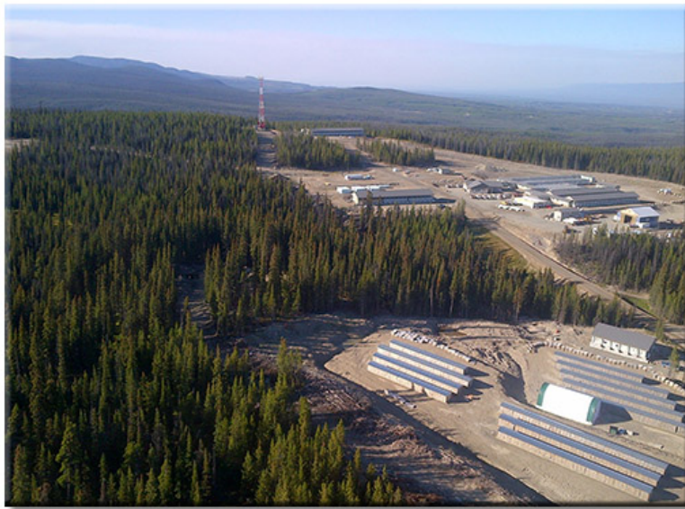
Photo ES 1: Aerial View of Blackwater Exploration Camp
