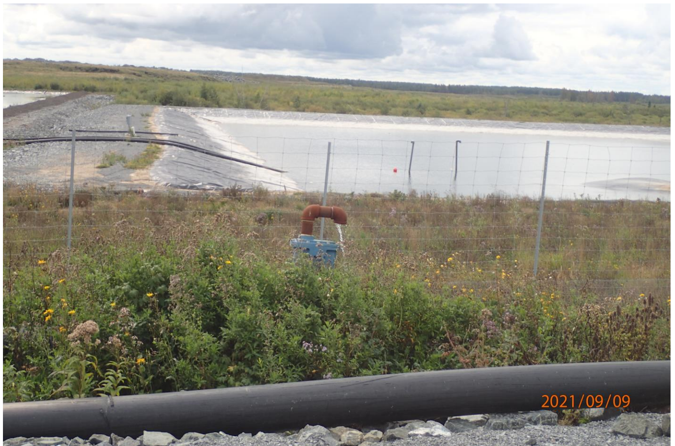
Photo 1: Leaking valve.
