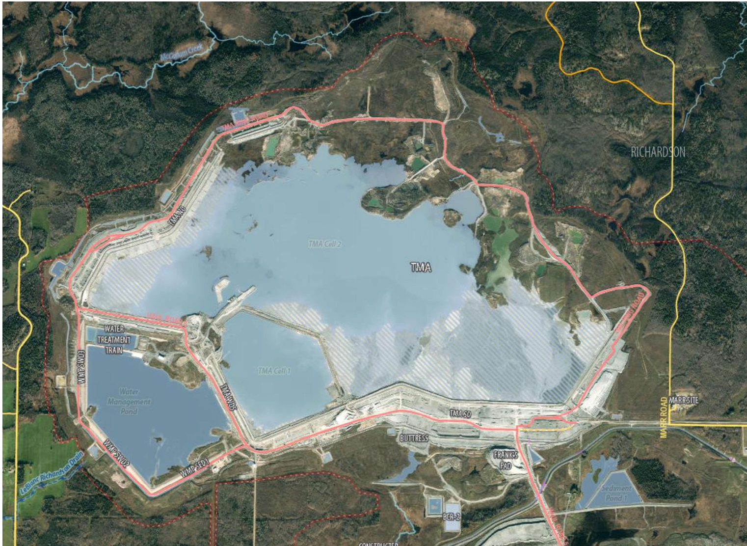
Figure 4- 1: Plan View of WMP, TMA and Associated Structure (Aug. 2021)
