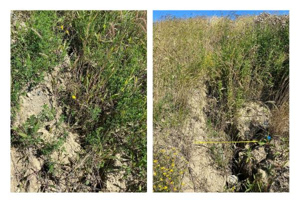
Figure 4: South Slope Rill (left) and Gully (right) erosion.
