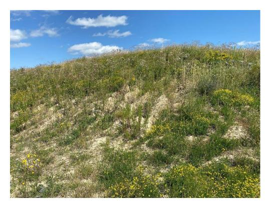
Figure 6: West Slope Rill erosion.
