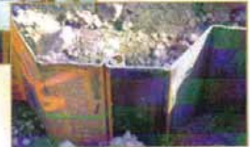
Waterloo Sealed Steel Sheet Pile Barrier
