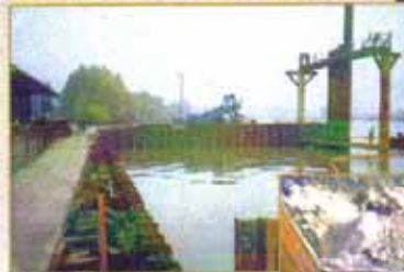
Steel Sheet Pile Barrier
