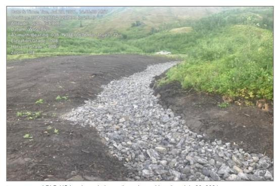
Photo 20: LBLD-US Laydown drainage through pond location, July 20, 2021.
