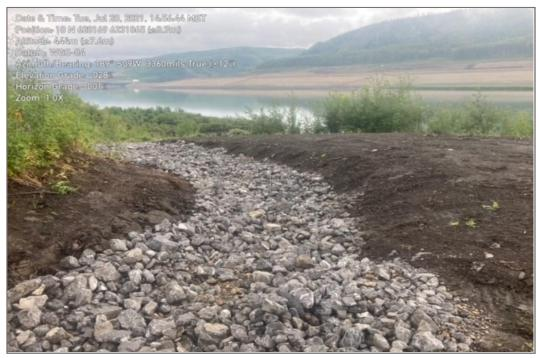
Photo 21: LBLD-DS Laydown drainage through pond location, July 20, 2021.
