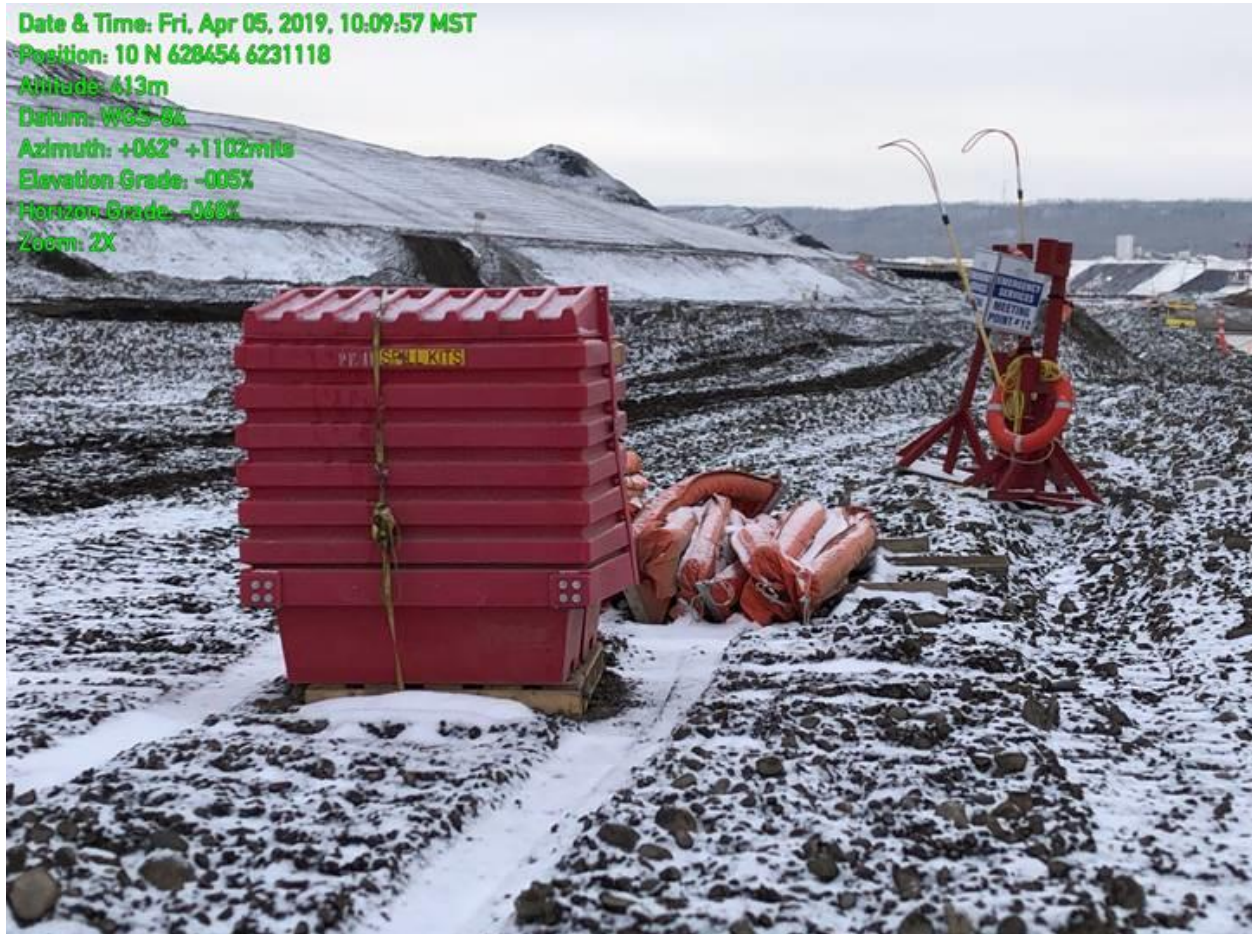
Figure 5. Absorbent and containment booms are on-site and available for deployment in the event of a spill at RSEM L5 (April 5, 2019).
