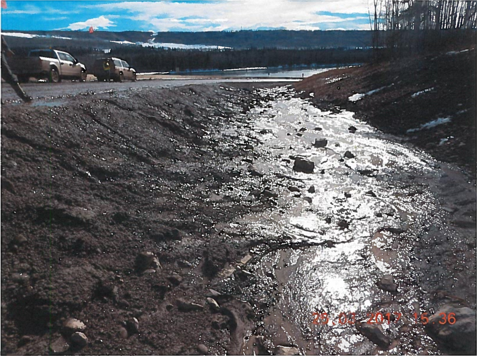
Figure 3: Sediment laden water flowing in ditch adjacent to River Road
