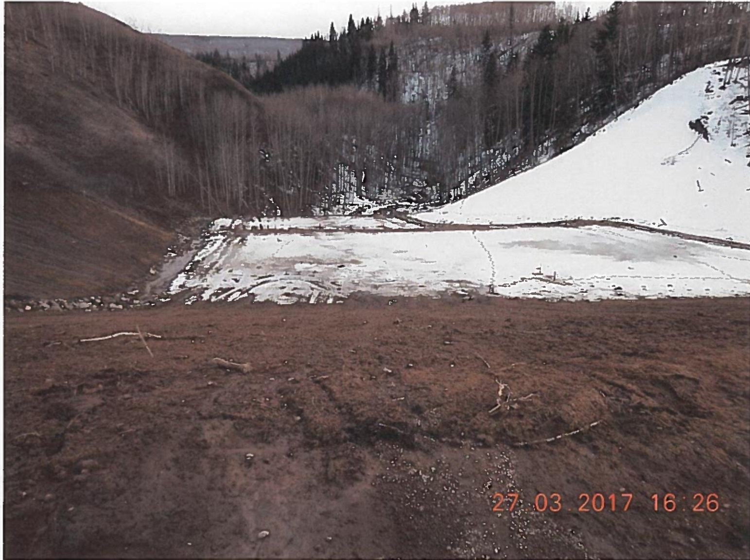
Figure 1: River Road Crossing upstream of Unnamed Creek 3
