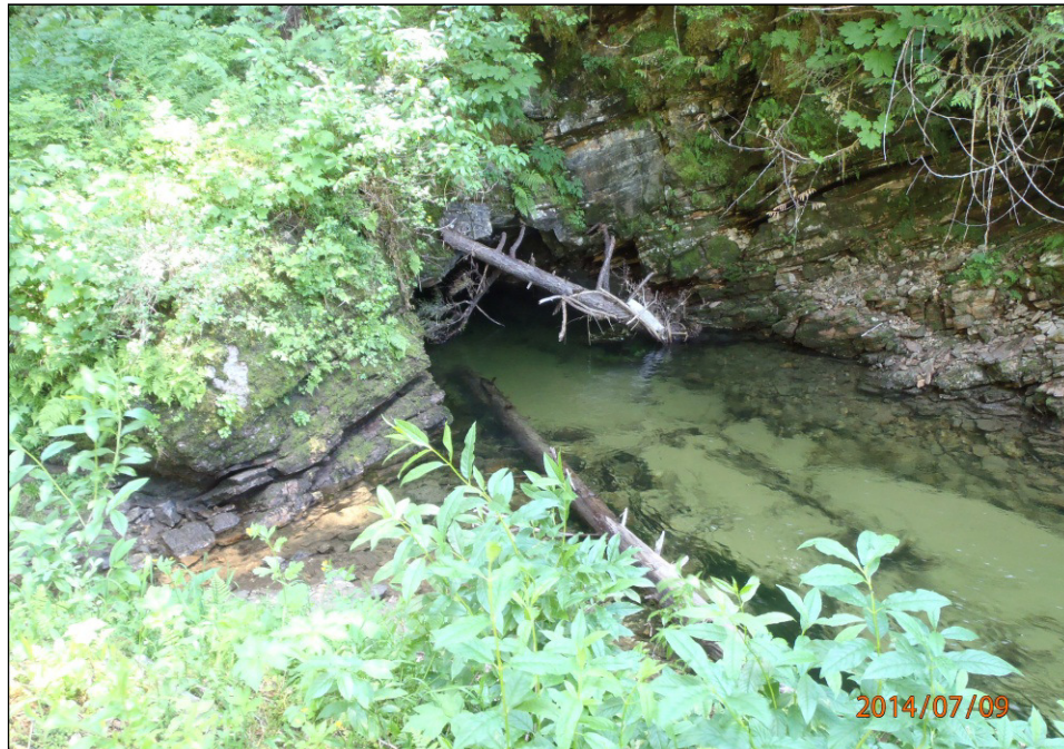
Plate 6.1-8. Upstream end of CN Rail water tunnel.
