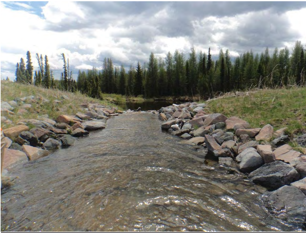
Figure 7. 25E Creek at outlet of 25E Lake (looking downstream) spring 2013
