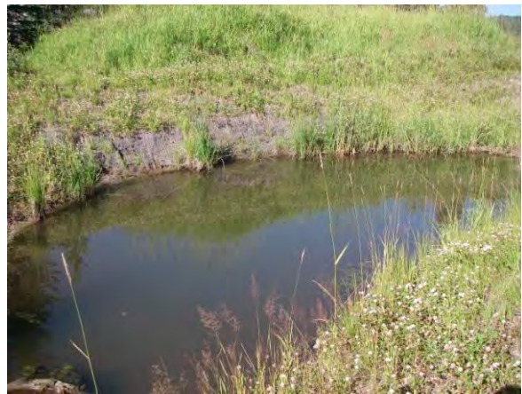
Photo 4. Looking at partially exposed bank along diversion channel.
