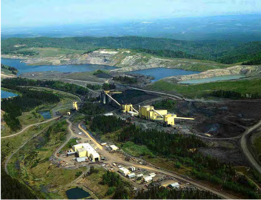
ESRD SIR2 Photo 17-1: Rock Fills within Tailings Pond
